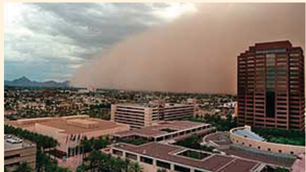
Dust storm, Phoenix, Arizona, August 19, 1999.
