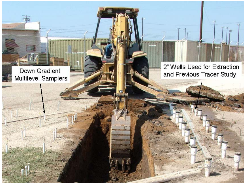
Figure 5. Removal of 1.2 m of the existing formation material to allow for the construction of the infiltration gallery.
