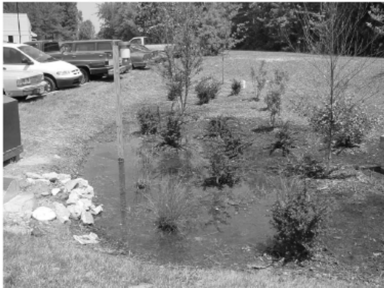
Figure 30. Bioretention cell C1 in Chapel Hill 8 months after construction (Hunt et al. , 2006).
