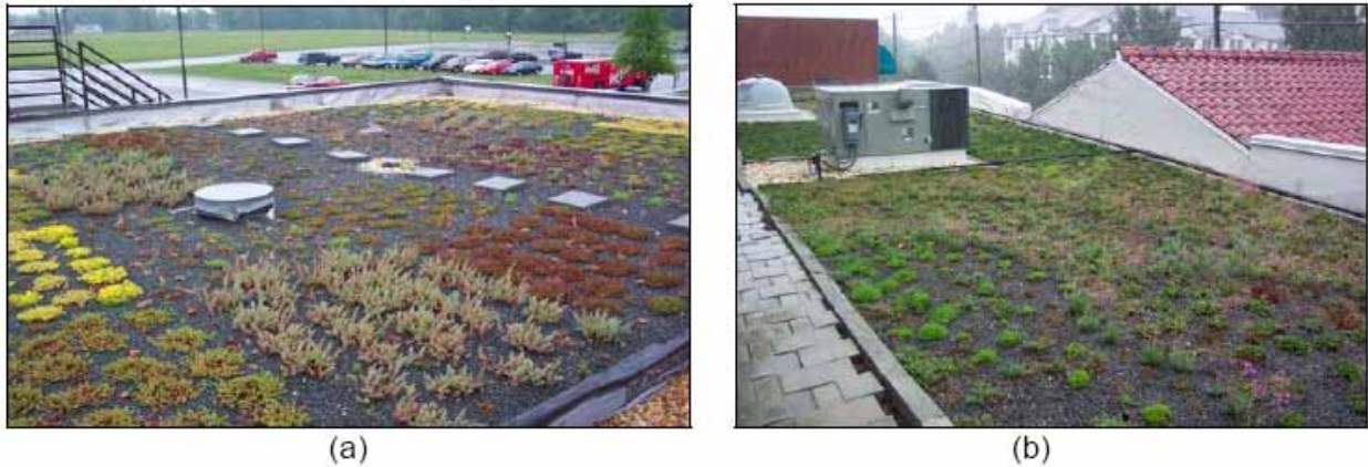
Figure 17. (a) WCC green roof in Goldsboro, NC (April 2003). (b) B&J green roof in Raleigh, NC (August 2004) (Moran et al. , 2006).
