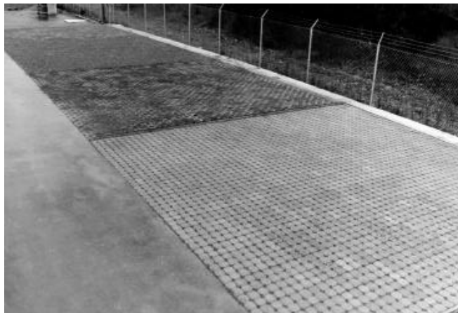
Figure 21. Reinforced gravel (top left), reinforced grass pavement (middle), and 90% impervious blocks with gravel (U.S. Environmental Protection Agency, 2000).
