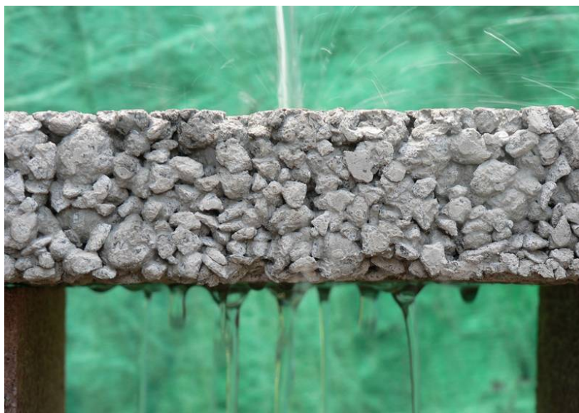
Figure 23. An example of a permeable pavement infiltration.
