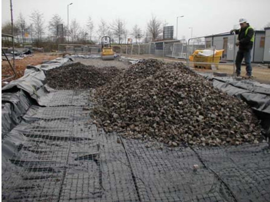
Figure 22. An example of a tanked permeable pavement system being built (Frederico, 2006).
