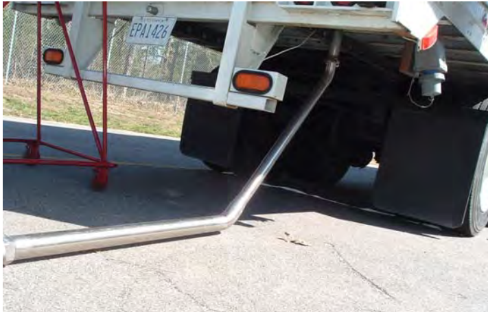
Figure 2-3. Sample line enters DEAL floor downstream of horizontal slipjoint and two 45° bends.
