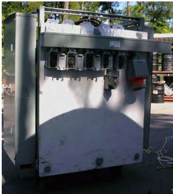
Figure 3-1. Electrical power skid used during APEX-2 and APEX-3.
