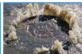
Aging Water Infrastructure
