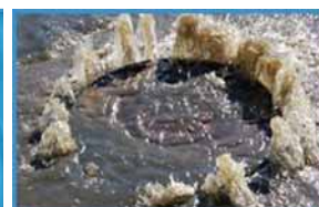
Aging Water Infrastructure
