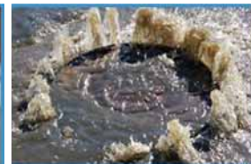
Aging Water Infrastructure
