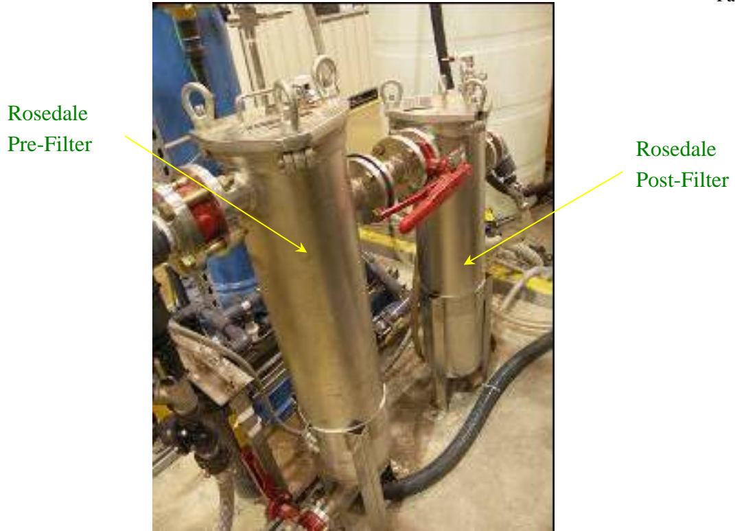
Figure 2-5. Rosedale PS 740 Filter Setup at the T&E Facility
