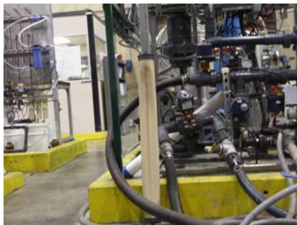
Figure 3-16. Deformed UF Filter
