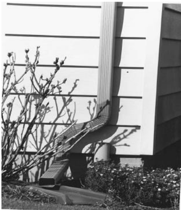
(Figure No. 3) Typical Residential Downspout Disconnection
