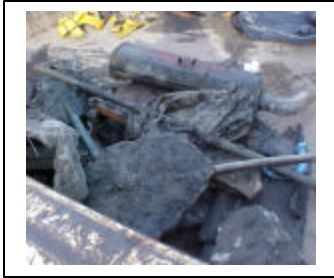
Figures 15, 16. Left, muffler and concrete pieces captured in a CDS unit during a rain storm. Right, trash, mostly plastics, removed by the same CDS unit (Continuous Deflective Separation). This CDS unit receives runoff from the City's highly congested downtown area, rich in pedestrians, visitors, trendy shops and restaurants, and the weekly Farmer's Market.
