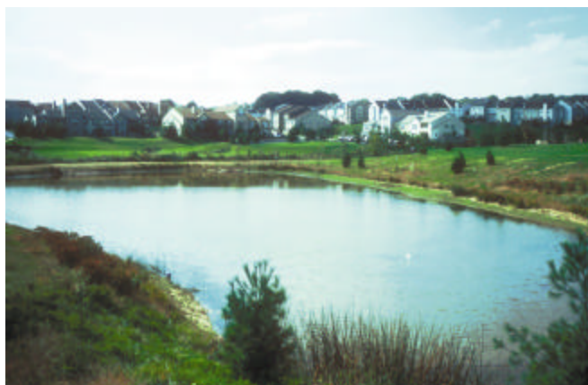
Figure 3a: 2-foot deep pond in Montgomery County Maryland (illustrating open water where a shallow marsh should be present)
