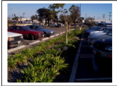
Figure 7, 8. On left, biofilter/swale system in parking lot of a school receives all runoff. For almost all storms, all runoff remains onsite for infiltration. On right, permeable pavers in a parking lot of a business allows runoff to infiltrate instead of run off into the street.
