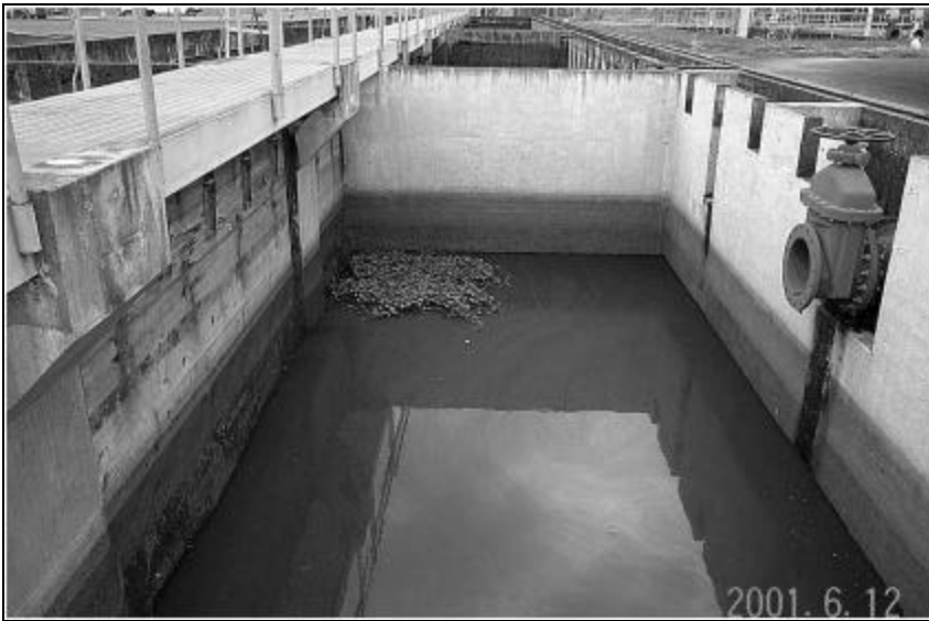
Figure 1 Photograph shows pennywort growing in the first cell of Portland's Vactor© waste decant tank. About three months after its initial introduction into the tank, the pennywort has formed a dense colony about 2.5 m square.
