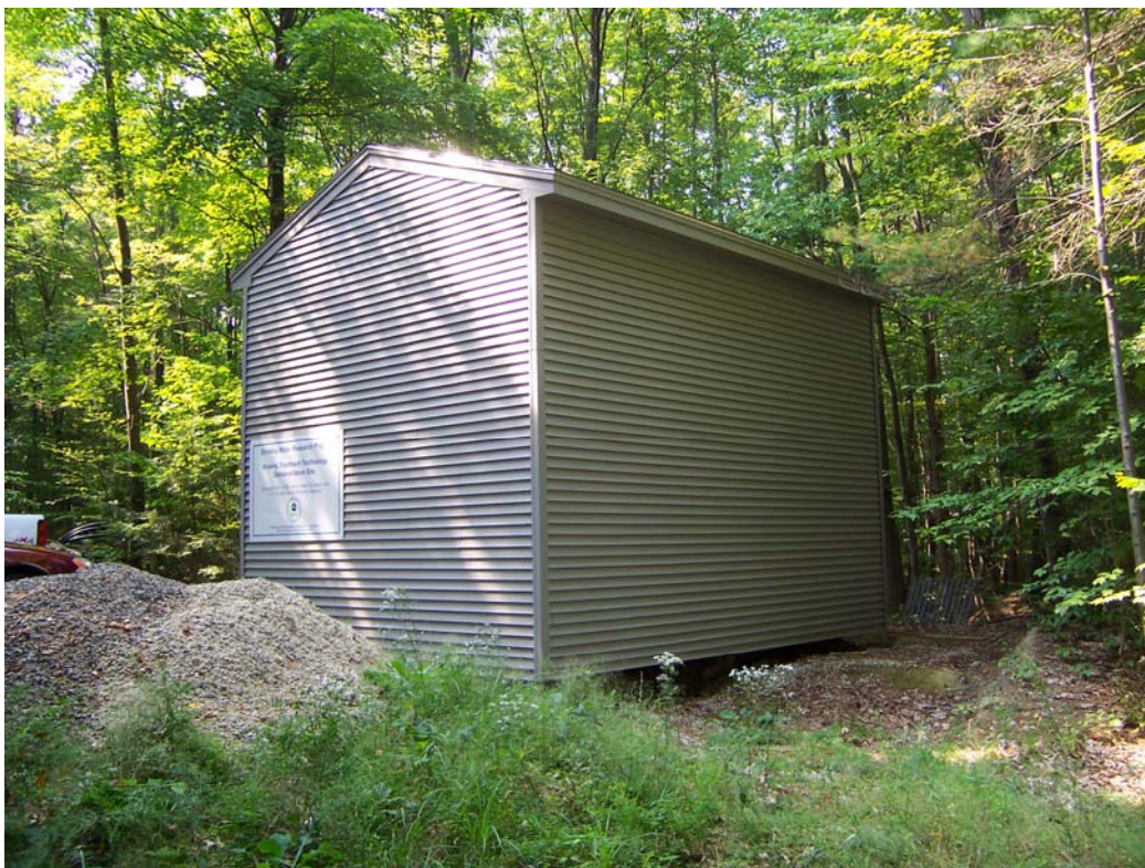
Figure 4-7. New Treatment Building Addition
