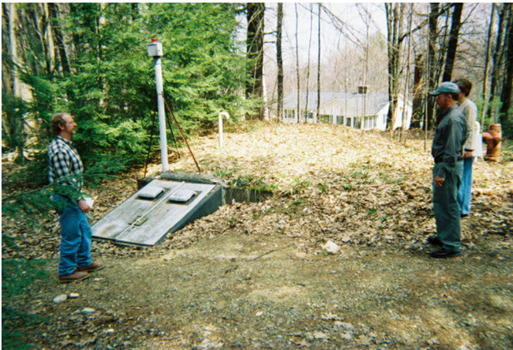
Figure 4-1. Existing Underground Treatment and Control Structure
