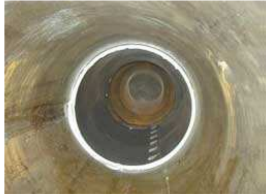
Figure 3-3. Link-Pipe 12 inch Pressure-Seal
