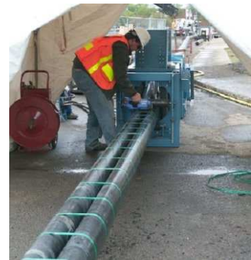
Figure 3-16. PolyFold™ Banding
