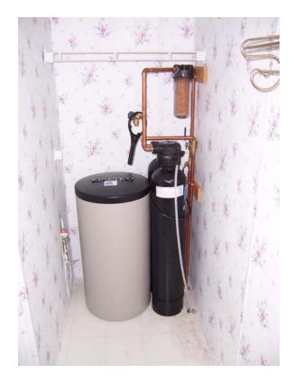
Figure 4-5. Kinetico Model 2060s Water Softener
