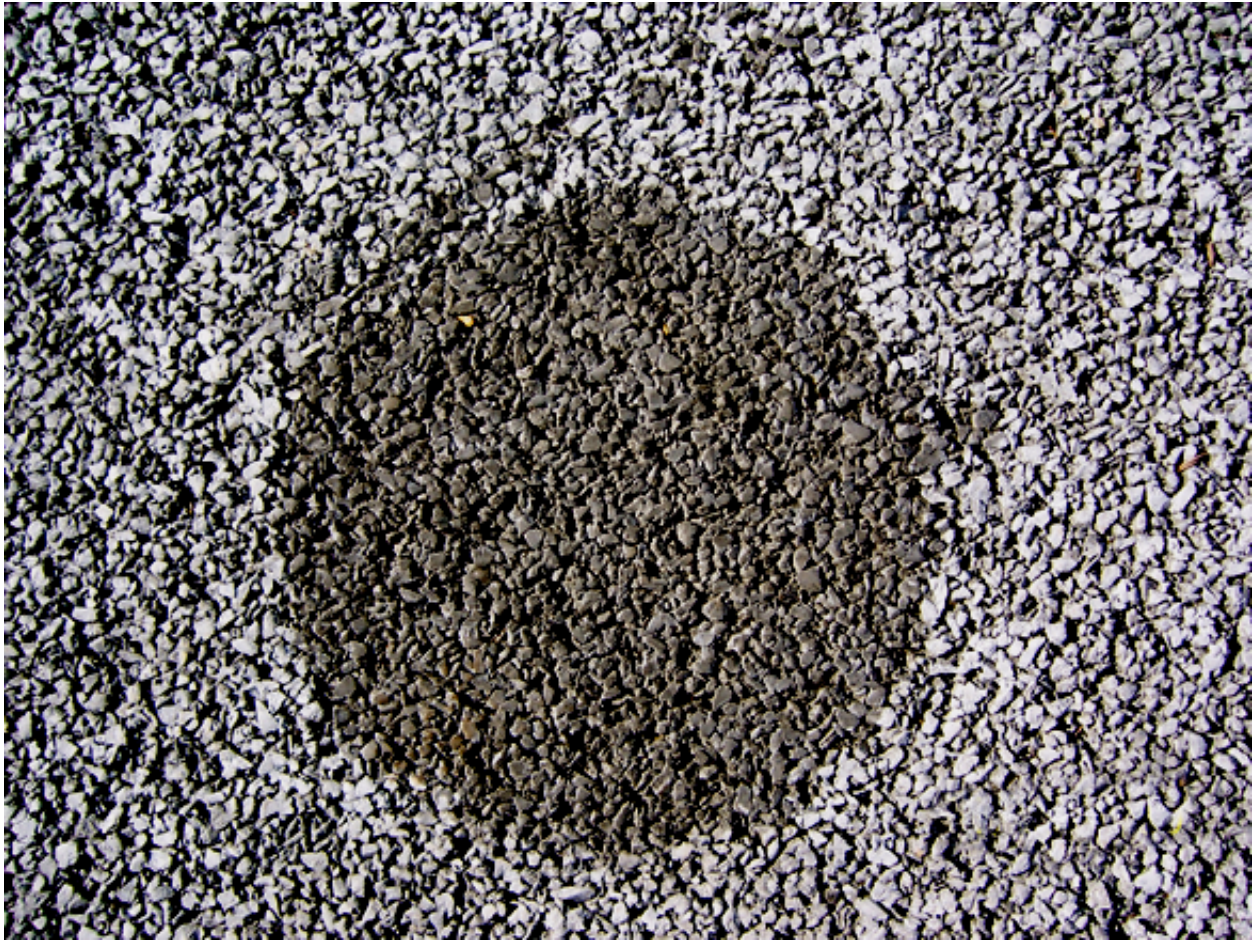
Figure 6. The wetted area after removing the test apparatus shows the limited leakage through the seal formed by the compressed Neoprene sheeting.
