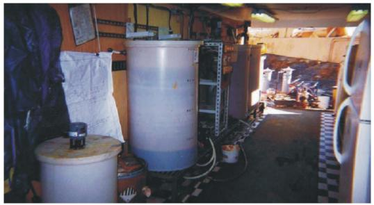
Figure 1-3. Ferrihydrite adsorption process in MWTP demonstration trailer.
