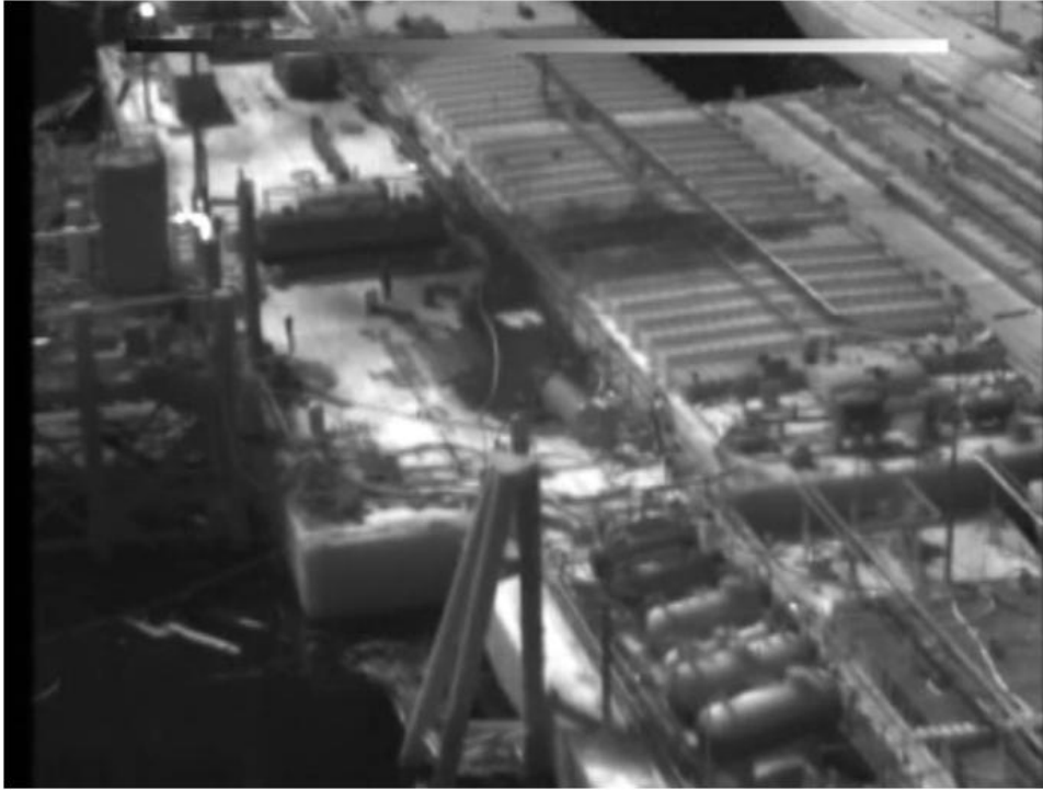
Figure B-3. Leak from Barge A14
