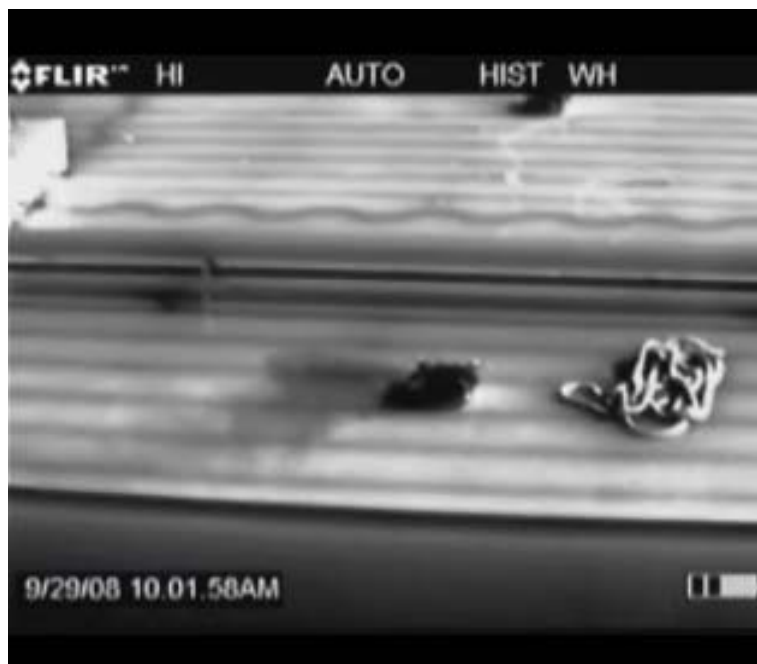
Figure 3-17. Example #3 from LSI Ground Survey – Leaking Hatch on Barge L6- Total Mass Emission from Barge 0.415 g/s
