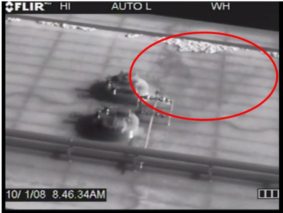
Figure E-6. Leak from Hatch 10/1
