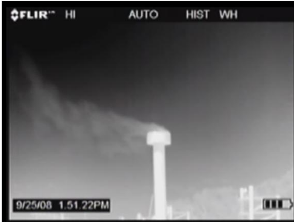
Figure D-13. Leak from Barge G3 (captured while onboard barge)
