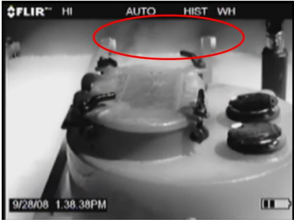
Figure D-27. Leak from Barge G8 (captured while onboard barge)
