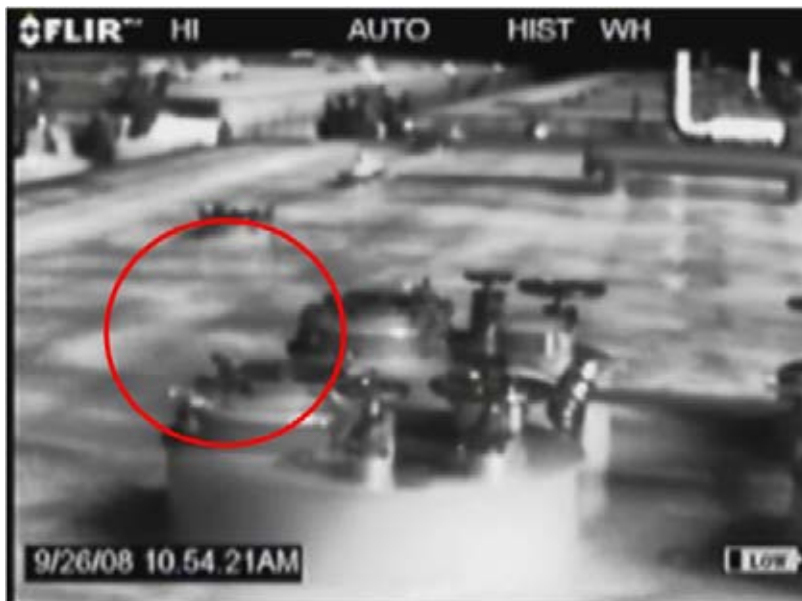
Figure 3-7. Leak from Ullage Hatch on Barge G4- Mass Leak 0.19 g/s
