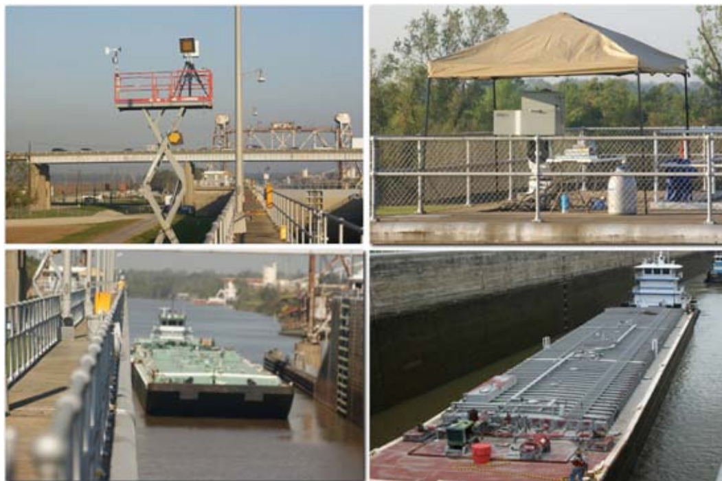
Figure 2-2. Images Illustrating OTM 10 Setup and Barges at the Port Allen Lock
