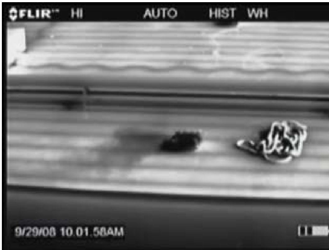
Figure 4-2. Screenshot from FLIR Camera Showing Leak from 9/29/ 2008, Event #2
