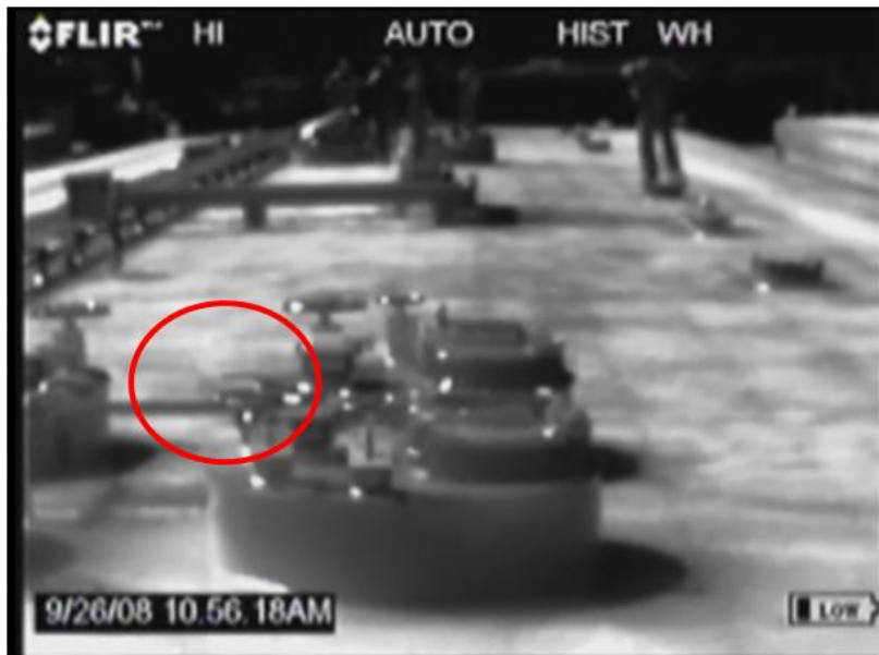
Figure 3-8. Leak from Ullage Hatch on Barge G4- Mass Leak 0.24 g/s
