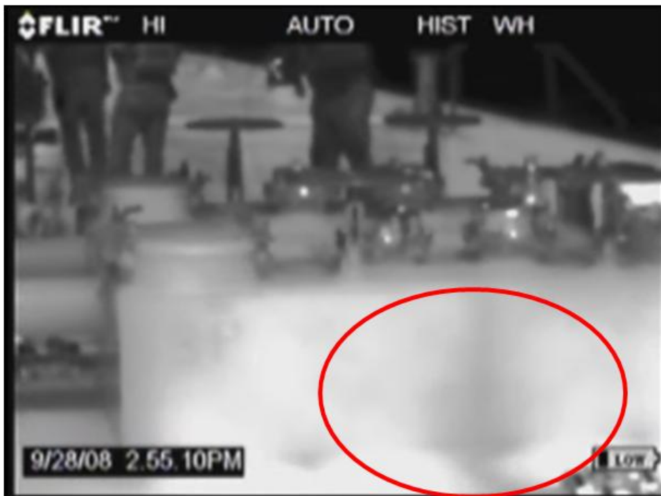
Figure D-34. Leak from Barge G8 (captured while onboard barge)
