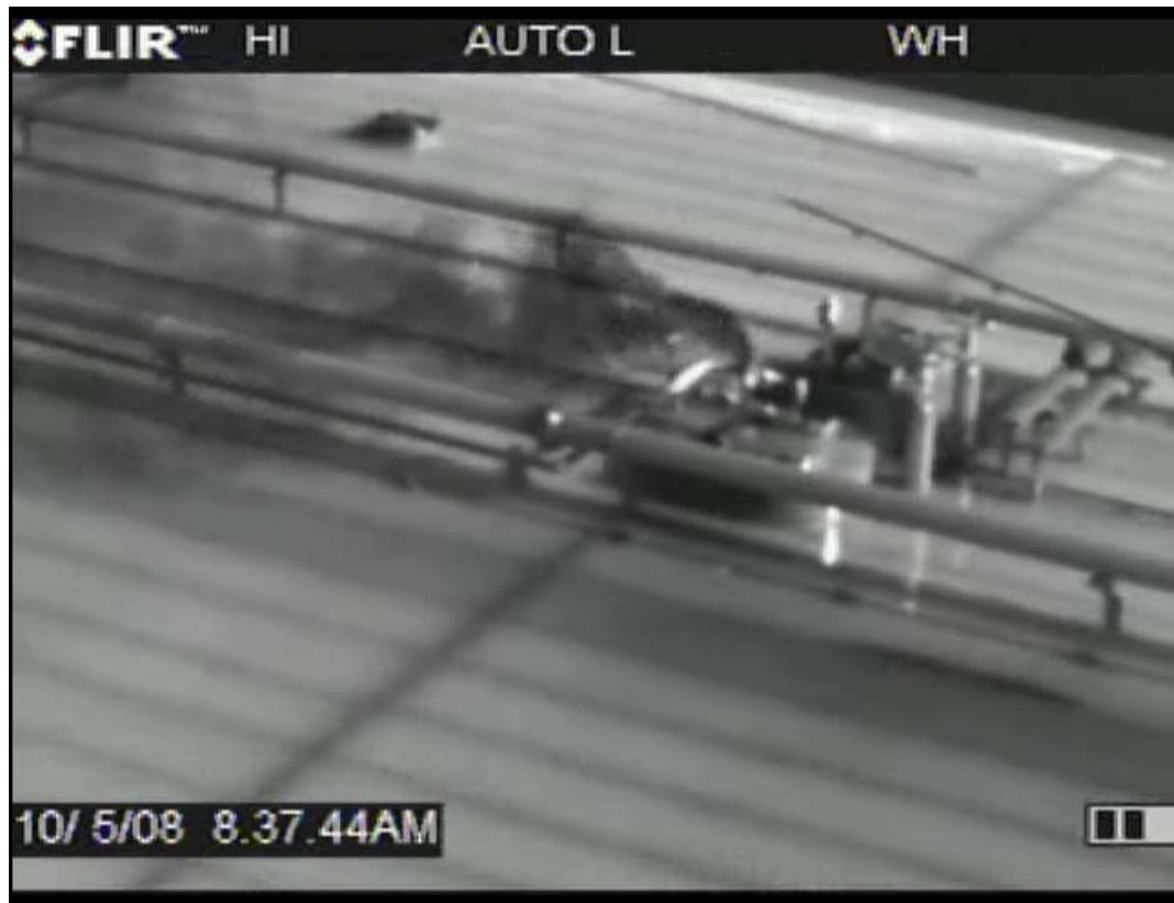
Figure 4-5. Screenshot from FLIR Camera Showing Leak from 10/5/ 2008, Event #1
