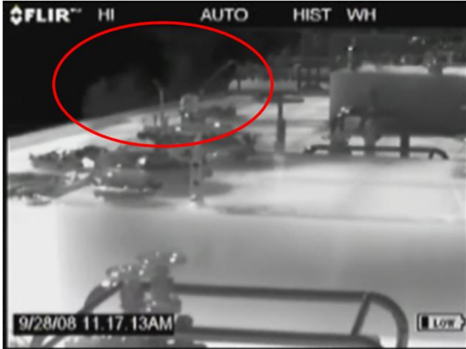
Figure D-24. Leak from Barge G7 (captured while onboard barge)
