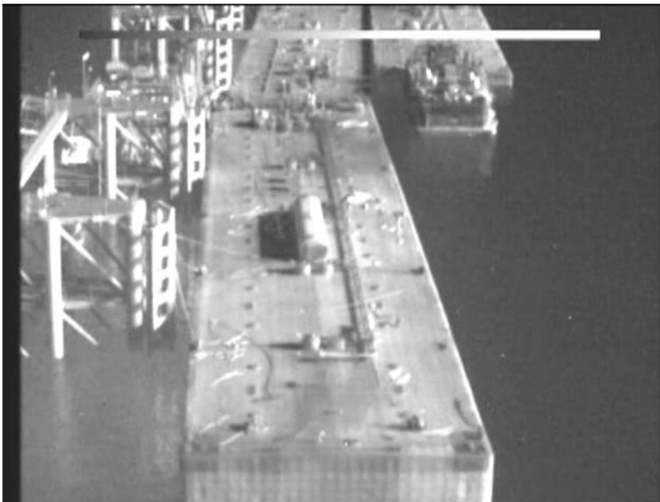
Figure B-6. Leak from Barge A19
