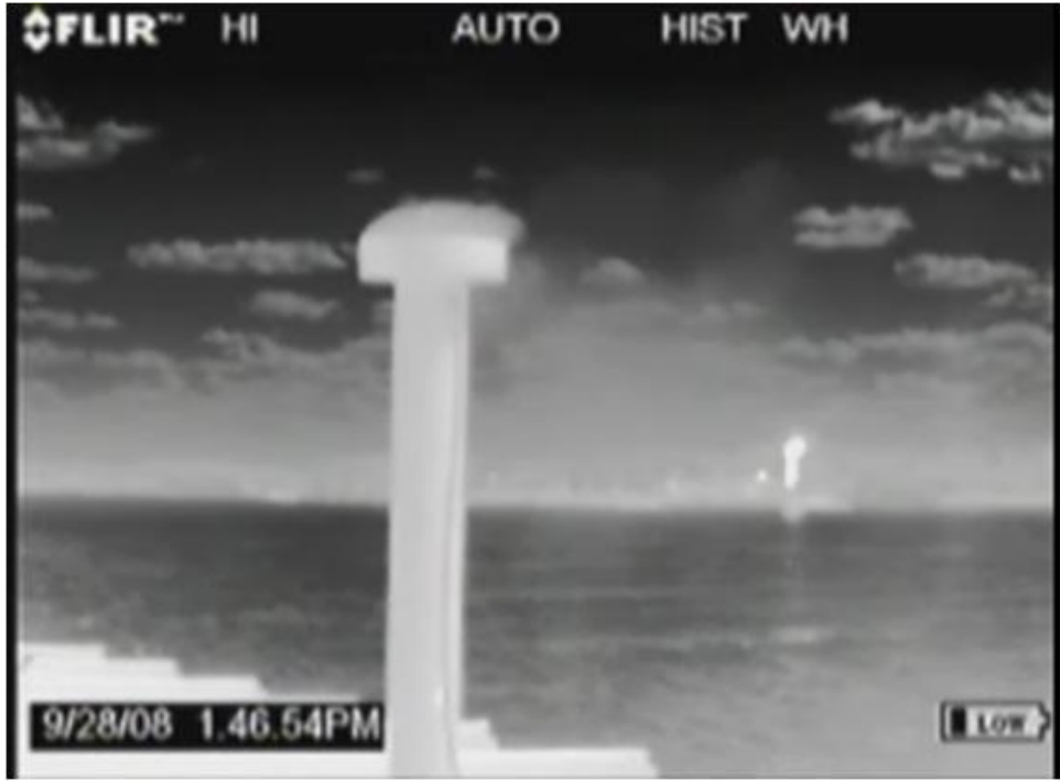
Figure D-30. Leak from Barge G8 (captured while onboard barge)
