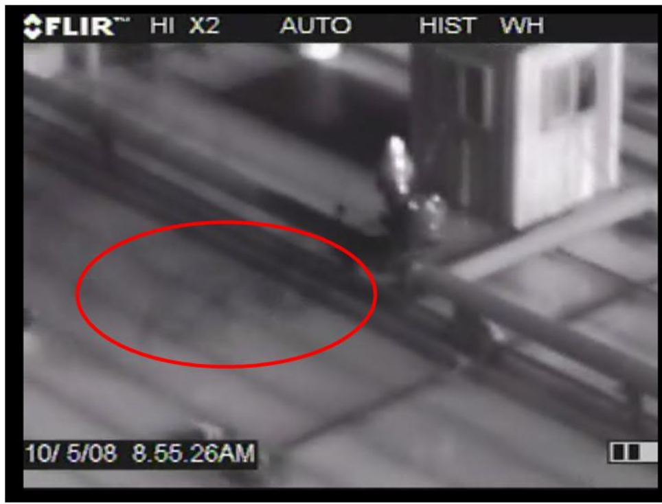
Figure E-15. Leak from Pipes 10/5
