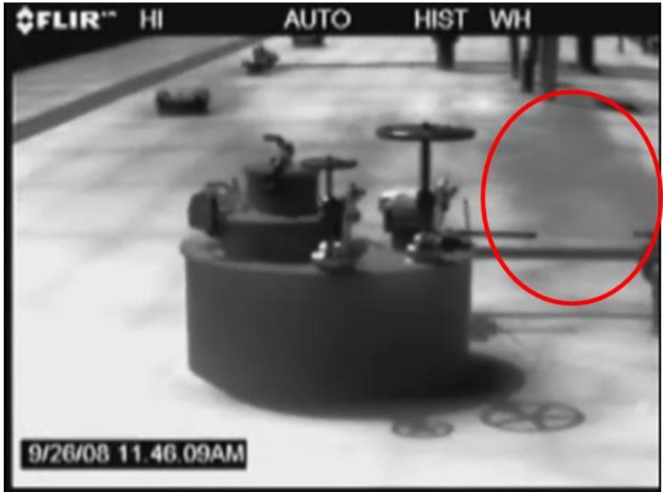
Figure D-17. Leak from Barge G5 (captured while onboard barge)
