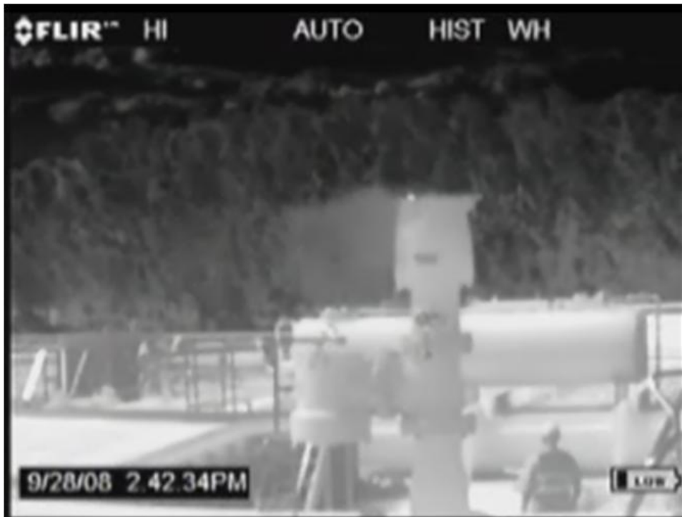
Figure D-31. Leak from Barge G8 (captured while onboard barge)
