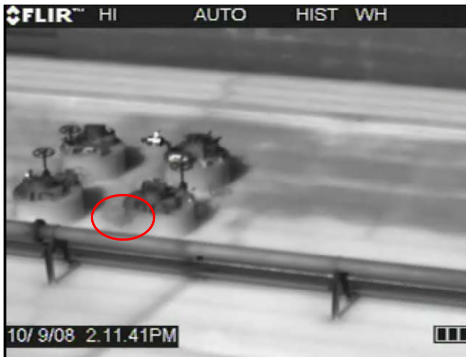
Figure 4-6. Screenshot from FLIR Camera Showing Leak from 10/9/ 2008, Event #7
