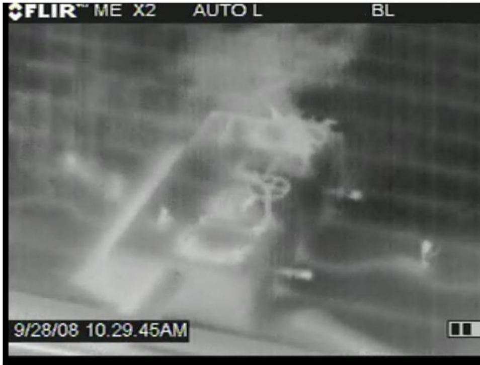
Figure E-1. Leak from Hatch 9/28
