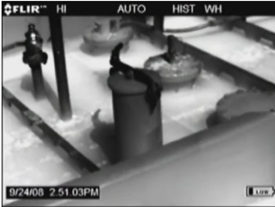
Figure D-6. Leak from Barge G2 (captured while onboard barge)
