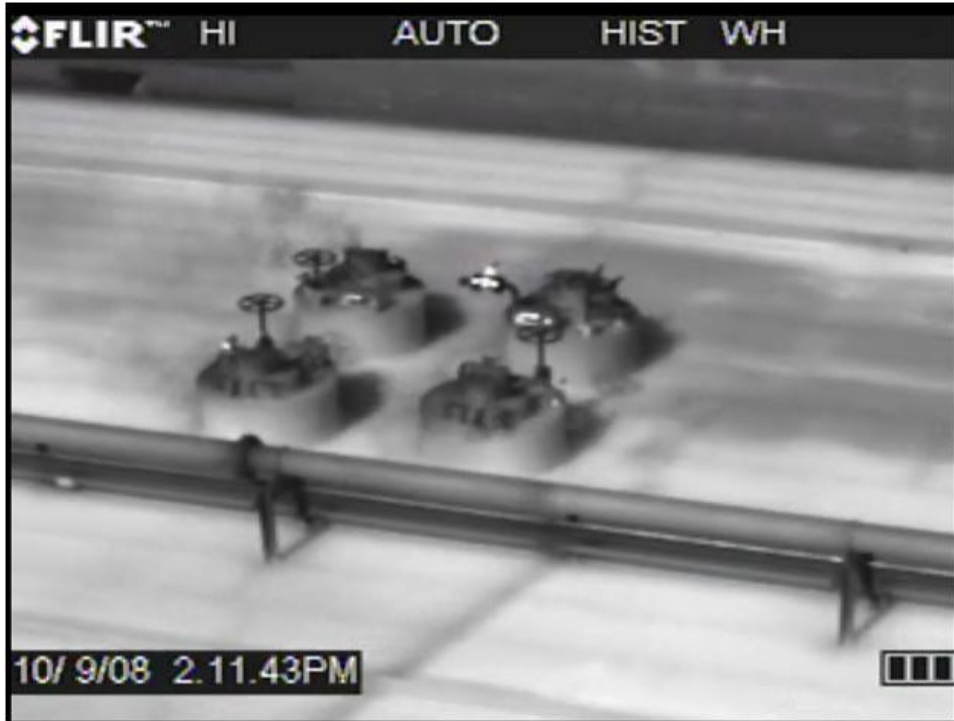
Figure E-17. Leak from Hatches 10/9
