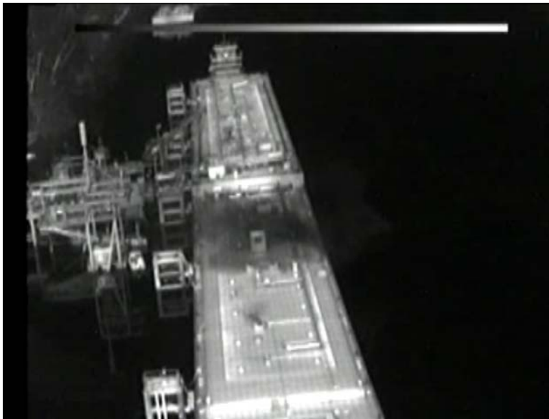
Figure 3-2. Example #2 from LSI Helicopter Survey – Leak from Vent Stack in Center of Barge A34
