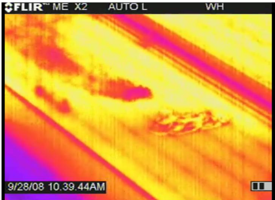
Figure E-2. Leak from Hatch 9/28
