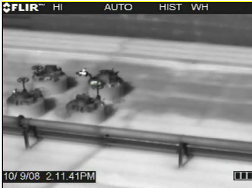
Figure G-10. Screenshot from FLIR Camera Showing Leak from 10/9/ 2008, Event #7
