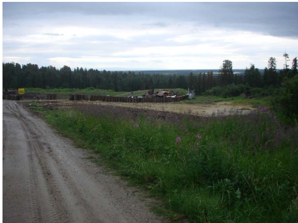
View of SW corner and toward natural drainage direction to the SE
