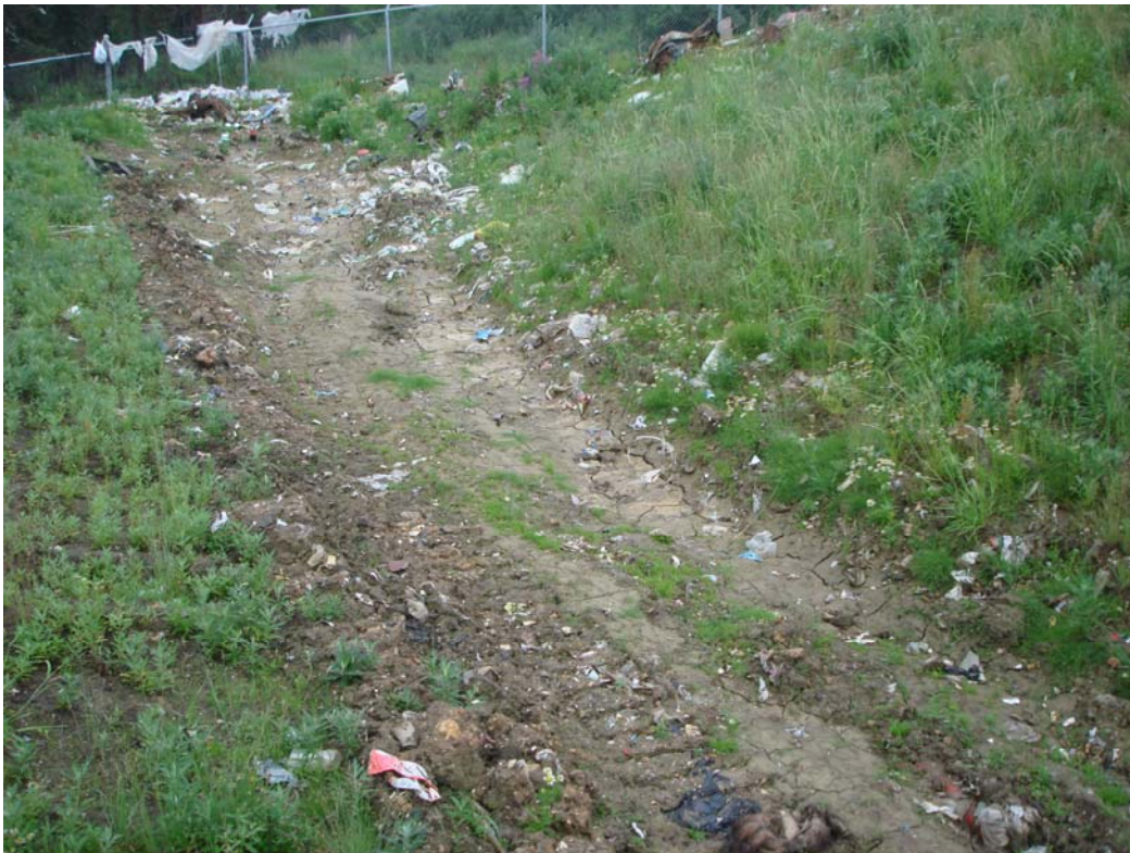
Exit of interior landfill drainage ditch by SE corner
