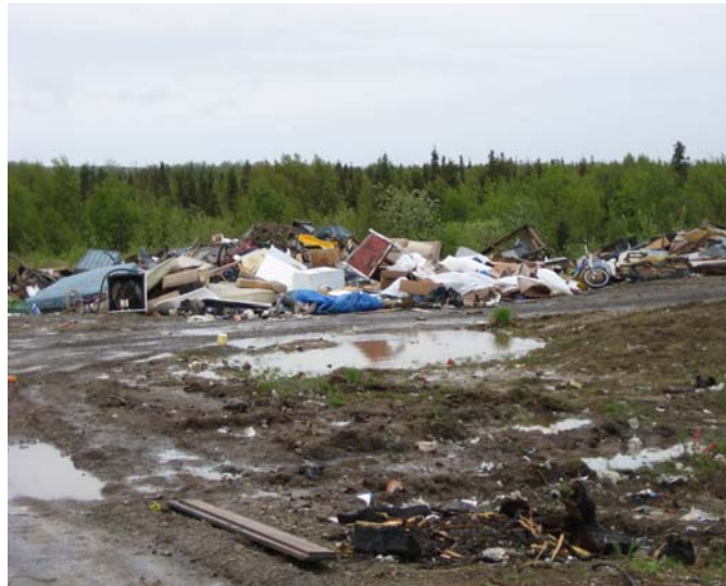
June 4, 2009, puddles after it rained Taken standing northeast looking northwest
