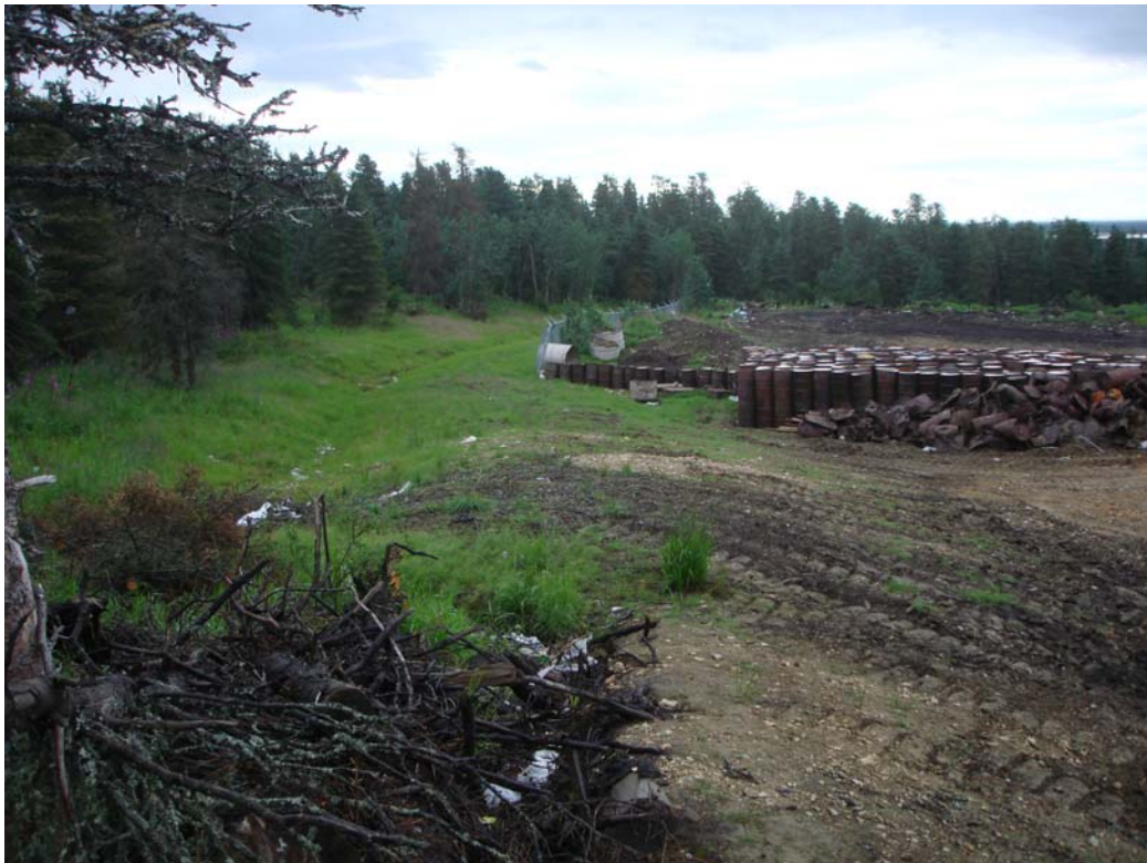
View of NW corner
