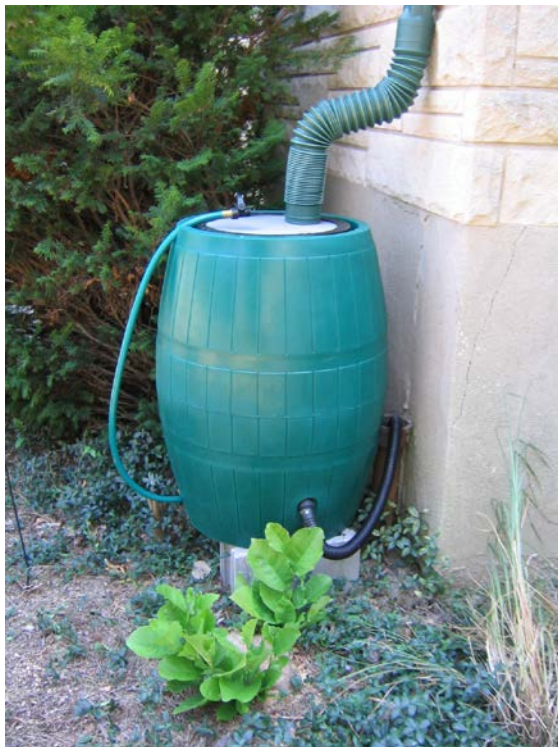
A Rainwater Catchment Device (Rain Barrel)
