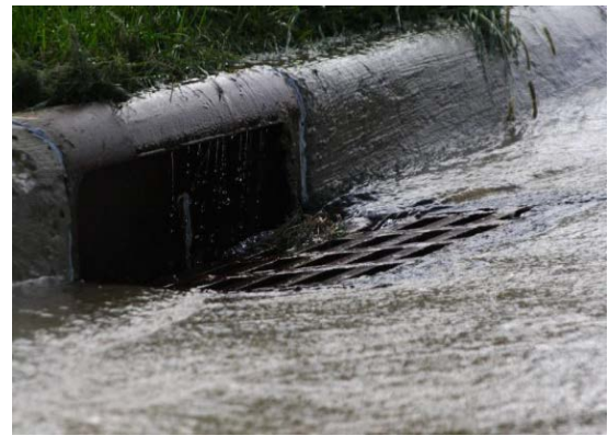
A Stormwater Collection Drain
