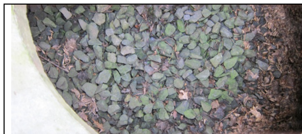
Dry well showing crushed stones at bottom with some minor lawn debris.
