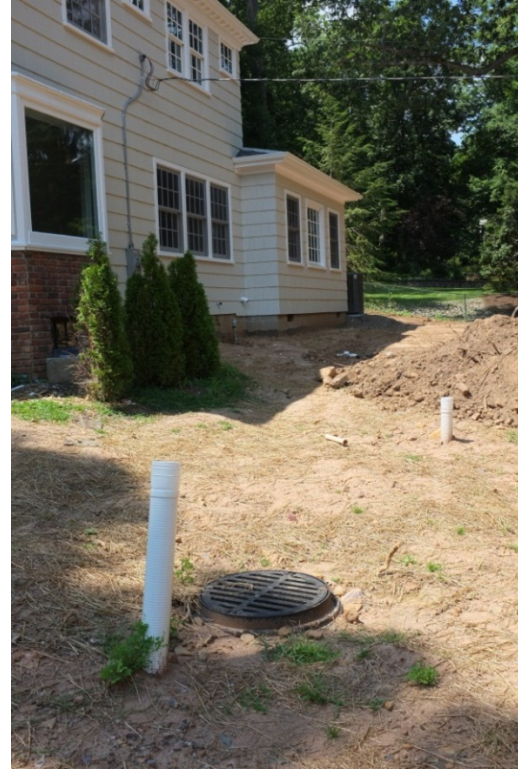
Frontyard dry well at new home used for water quality monitoring on Slope Drive open grating receives surface inflows in addition to roof runoff.
