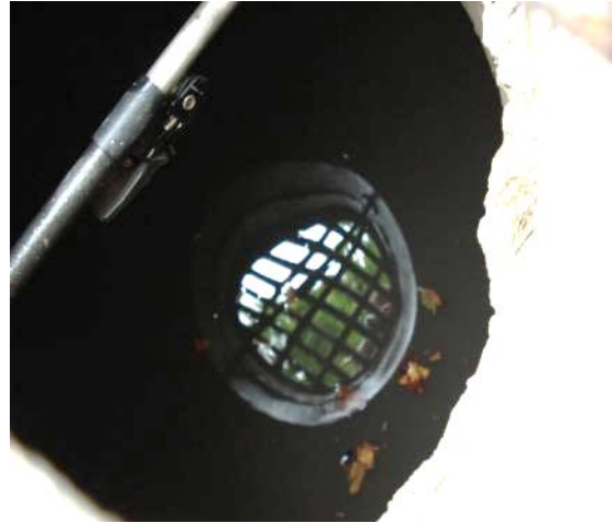
Dry well with standing water (383 Wyoming)
