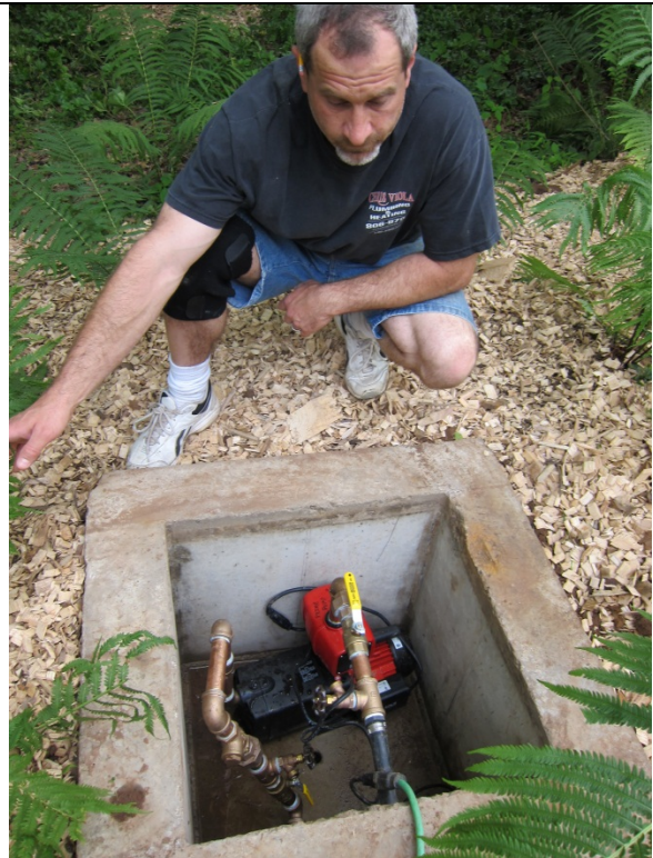
Cistern irrigation pump.
