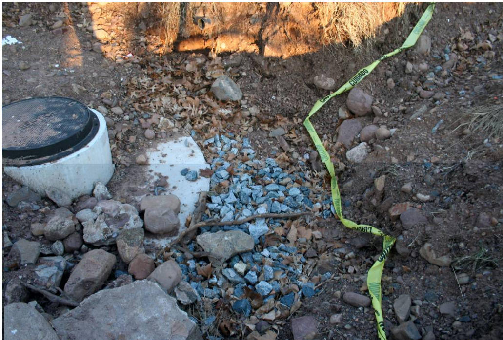
Figure 2-3. Installed dry well in Millburn, NJ, showing the surrounding blanket of crushed stone before completion of the backfilling (photo from Mel Singer).
