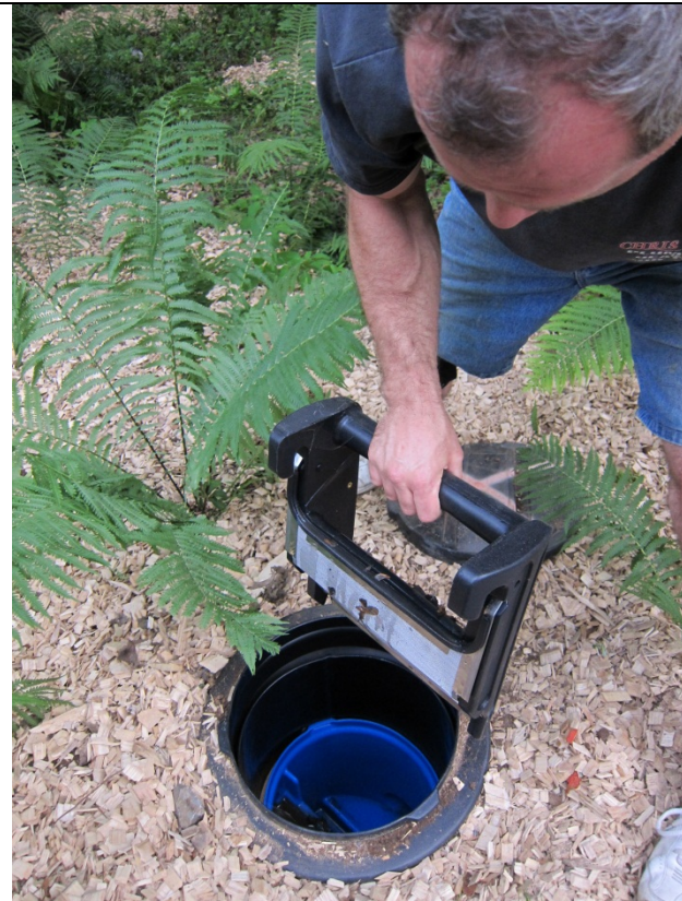
Cistern inlet filter.
