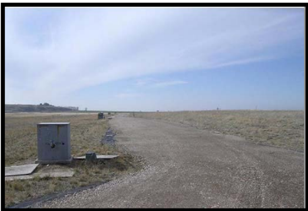
Fig. 5. A view of the Eastern Michaud Flats capped site
