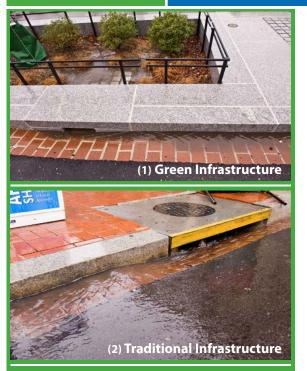
The National Stormwater Calculator shows users how land use decisions and green infrastructure controls affect the amount of stormwater runoff produced. Green infrastructure, such as the street planter and porous pavers shown in the image (1) above, promotes the natural movement of water within an ecosystem or watershed, instead of allowing it to wash into streets and down storm drains as shown in the traditional infrastructure image (2).
