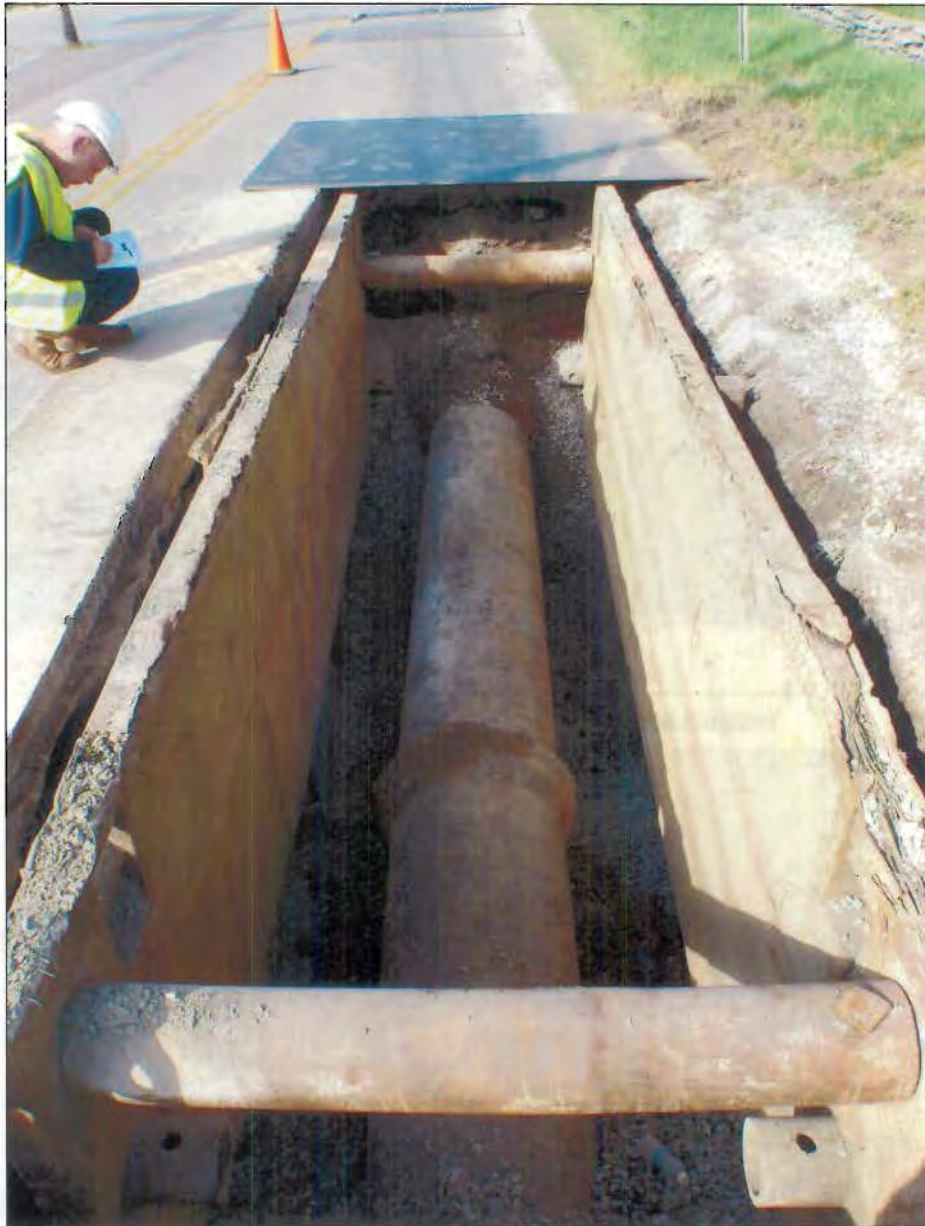
FIGURE A5.2 - PHOTOGRAPH OF PIPE IN EXCAVATION
