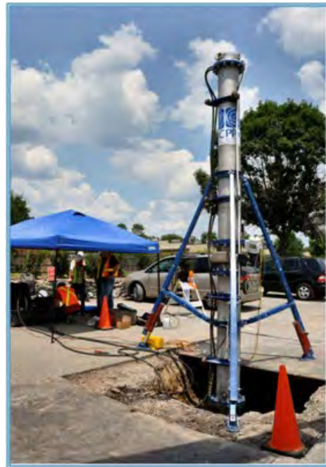
PipeDiver insertion tube setup at the launch site.
