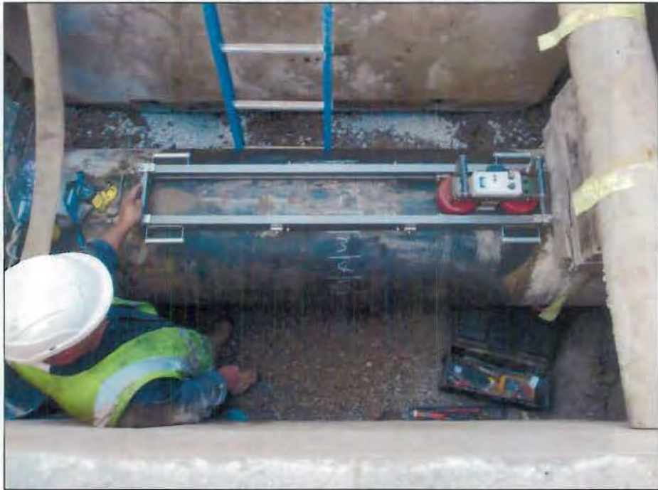
FIGURE A5.14 - PHOTOGRAPH OF MFL TOOL ON THE PIPE
