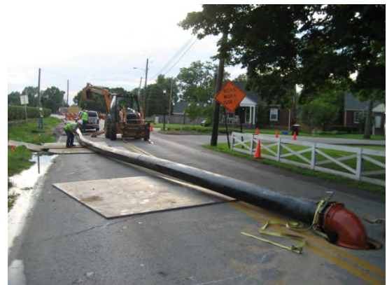
Figure 3-27. Test Pipe Discharge to Storm Sewer Configuration
