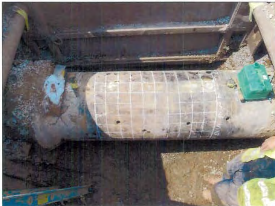
FIGURE A5.7 - PHOTOGRAPH OF COATING / CORROSION GRID
