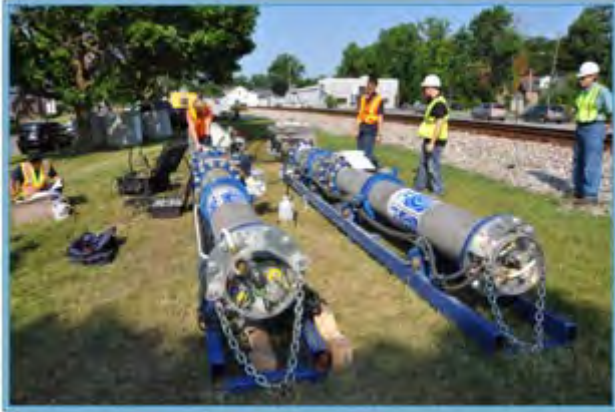
Preparing the PipeDiver insertion and retrieval tubes.
