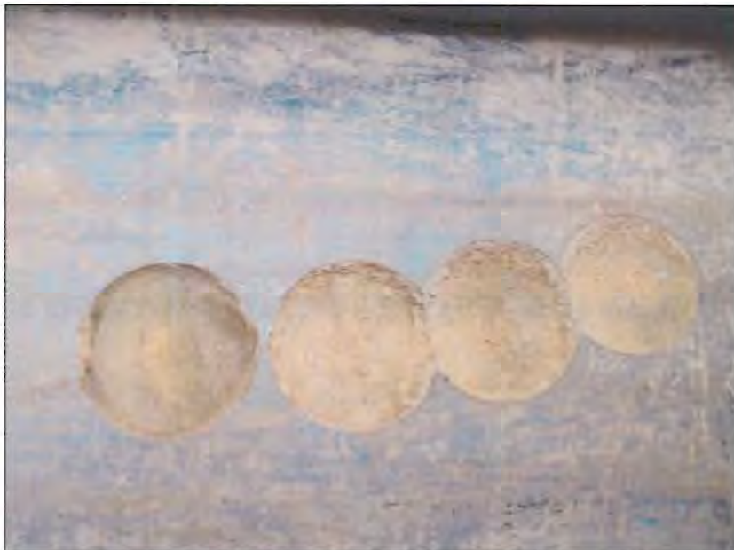
FIGURE 4.6 - MACHINED HEMISPHERICAL DEFECTS
