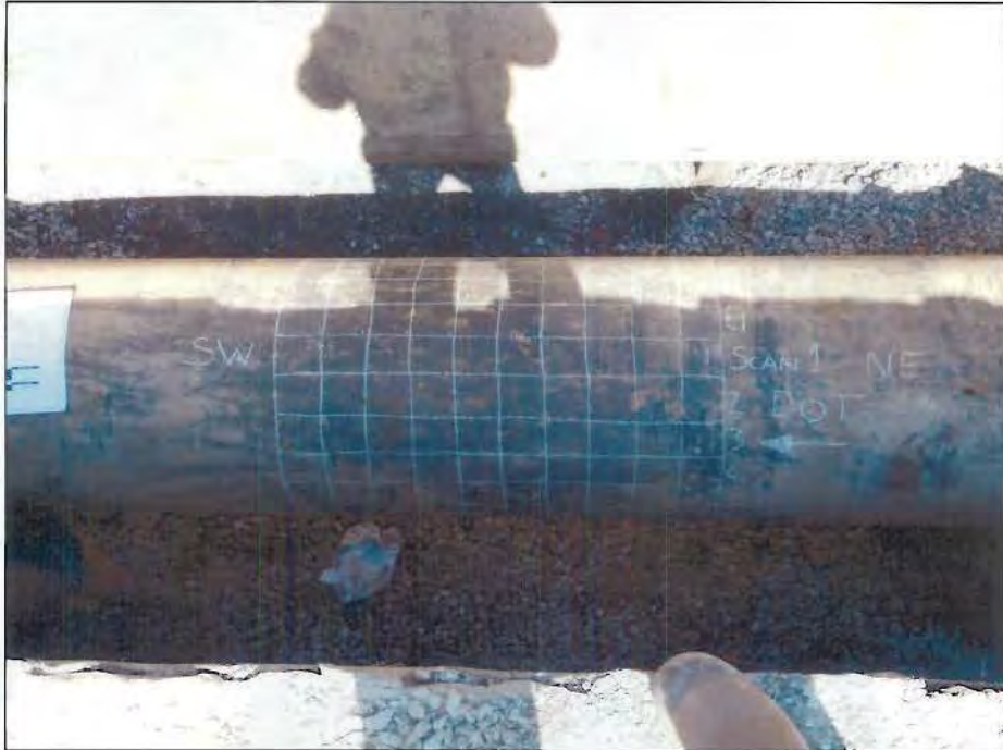
FIGURE A5.3 - PHOTOGRAPH OF COATING / CORROSION GRID
