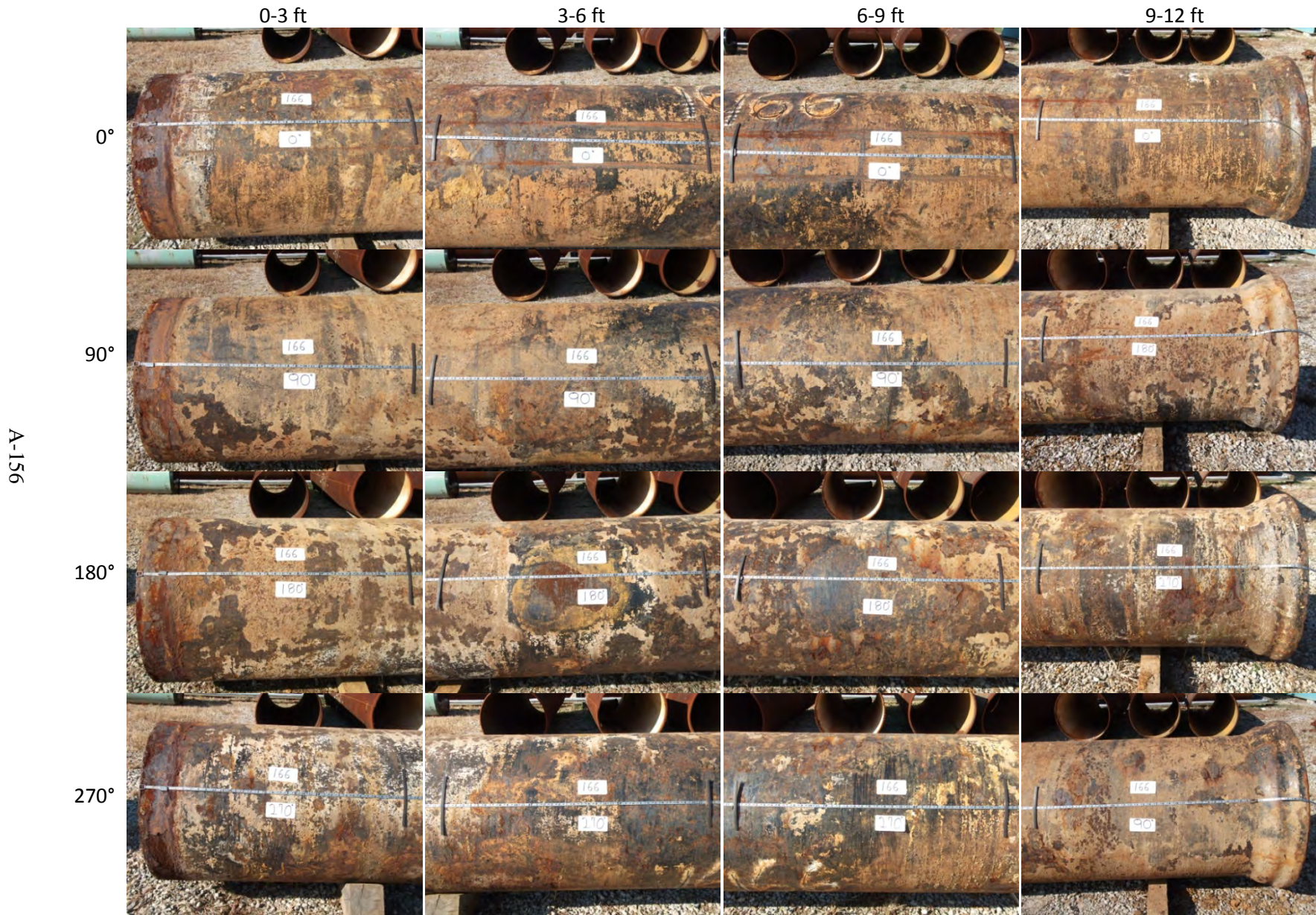
Figure A-166(1). Pipe 166 as Removed from Site
