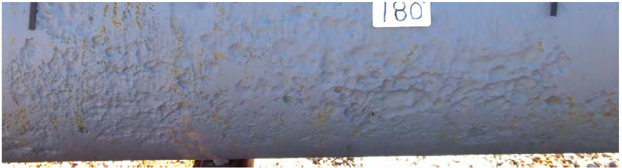
Figure 4-8. Photograph of Pipe 63
