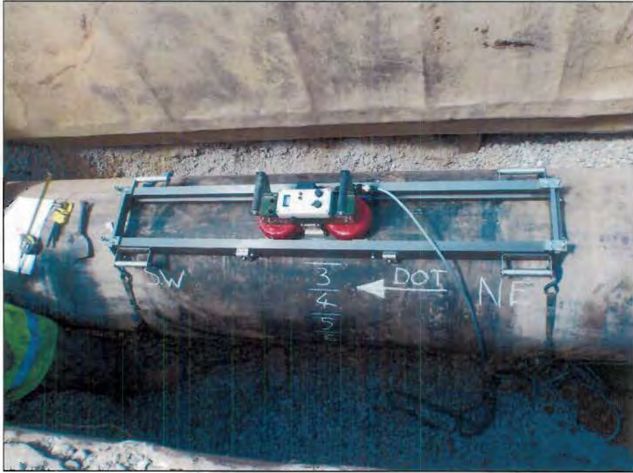
FIGURE A5.4 - PHOTOGRAPH OF MFL TOOL ON THE PIPE
