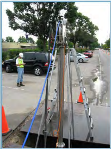
The Sahara insertion tube setup in Pit 1.
