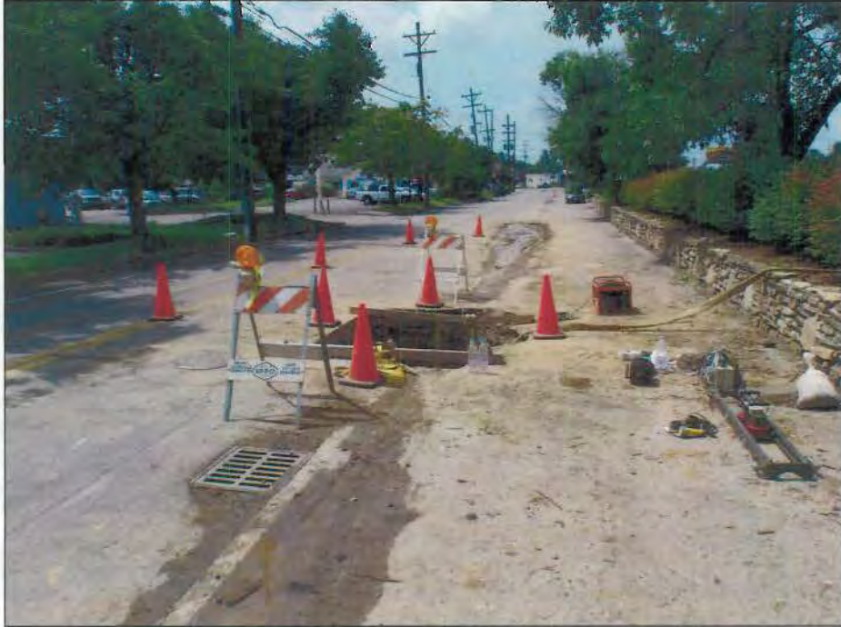
FIGURE A5.11 - PHOTOGRAPH OF EXCAVATION LOCATION
