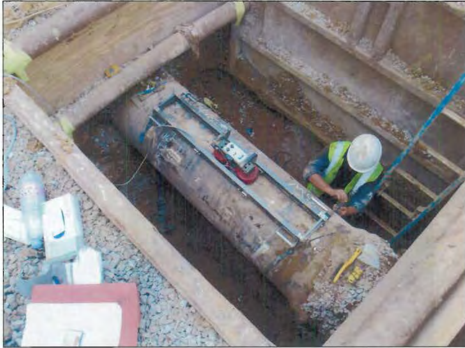
FIGURE A5.8 - PHOTOGRAPH OF MFL TOOL ON THE PIPE
