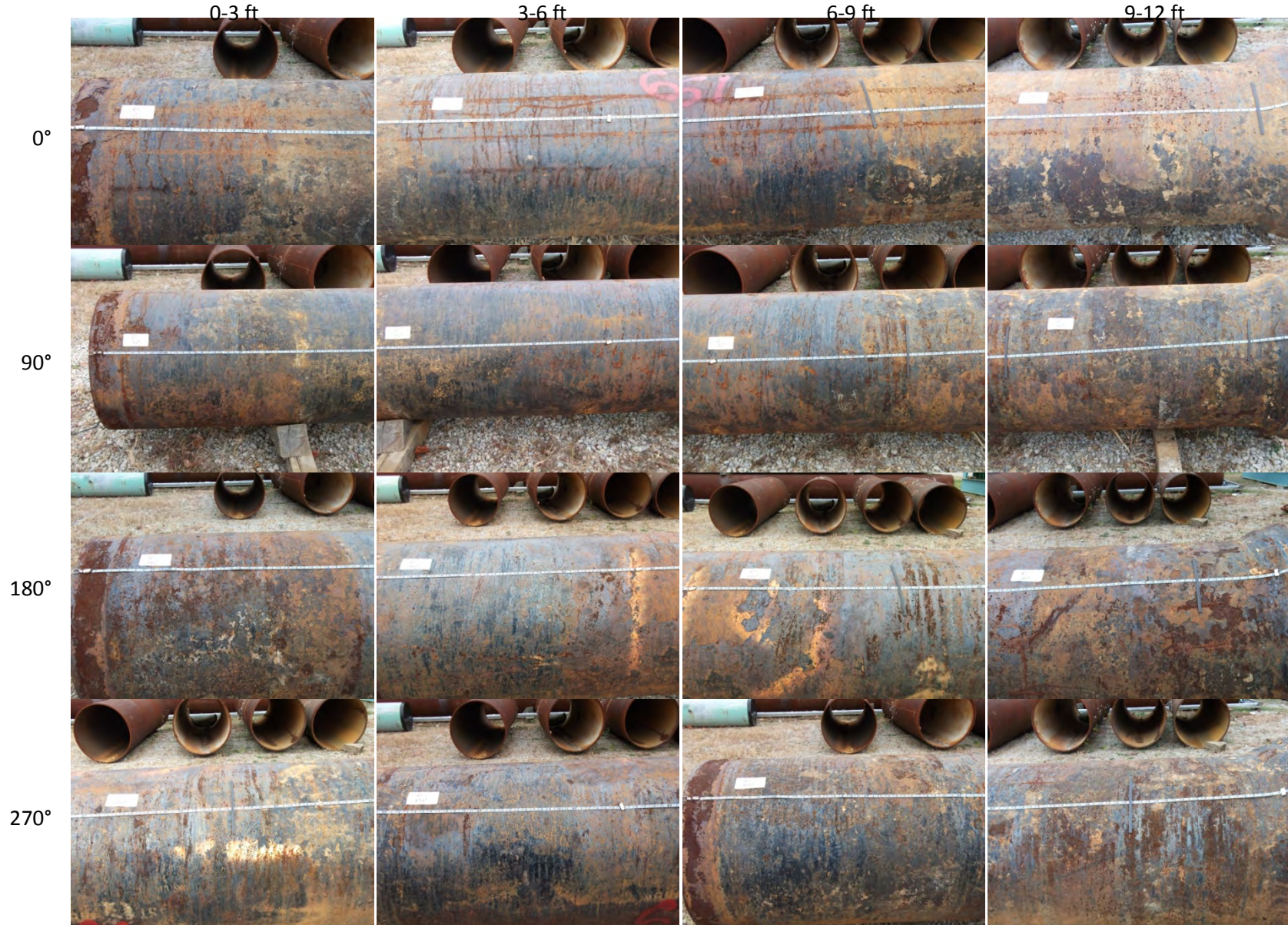
Figure A-61(1). Pipe 61 as Removed from Site
