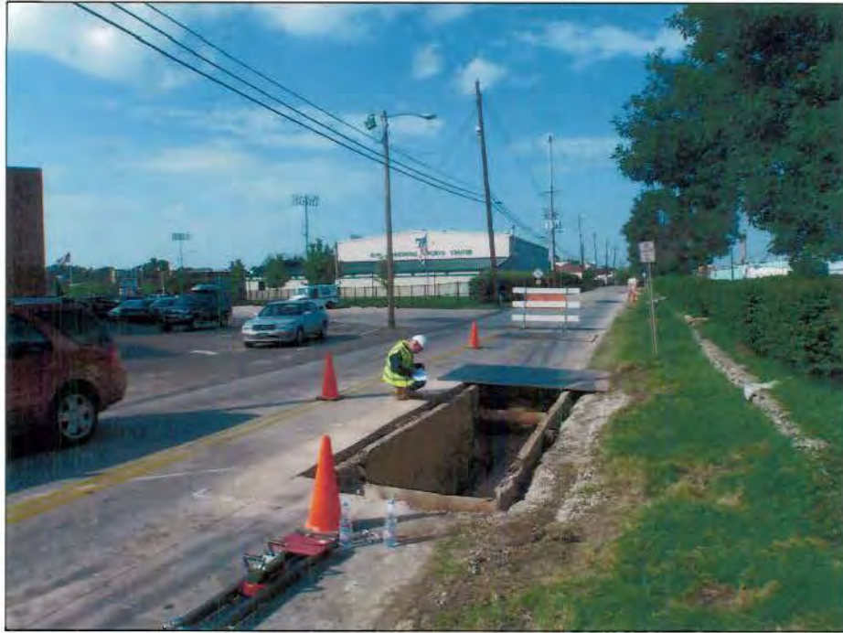
FIGURE A5.1 - PHOTOGRAPH OF EXCAVATION LOCATION
