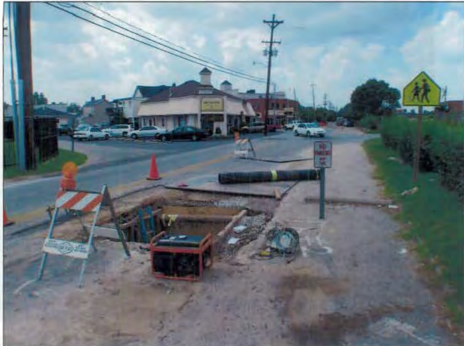
FIGURE A5.6 - PHOTOGRAPH OF EXCAVATION LOCATION
