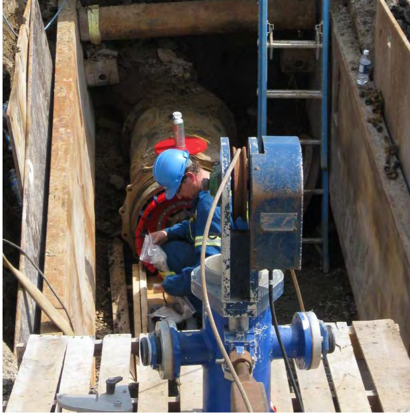
• Figure 3. Tool start position with hydrant adaptor and odometer wheel.
