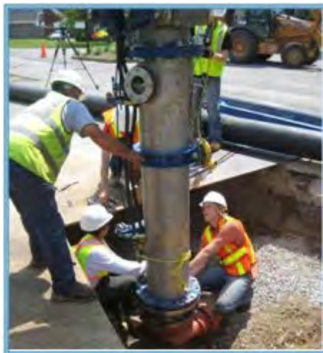
Attaching the PipeDiver extraction tube on the gate valve.
