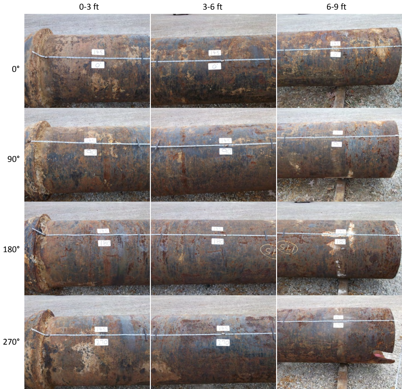
Figure A-145(1). Pipe 145 as Removed from Site
