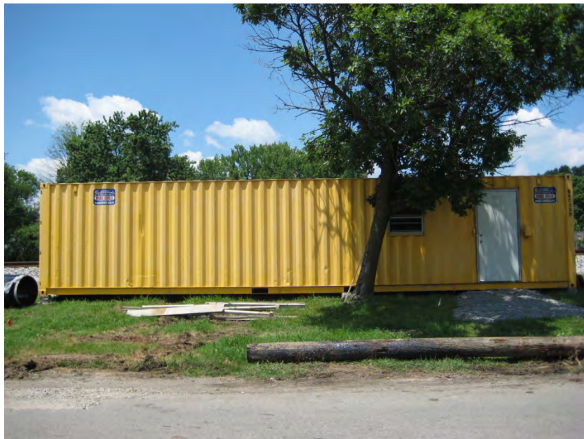
Figure 3-22. Construction Trailer for Equipment Storage and Work Space
