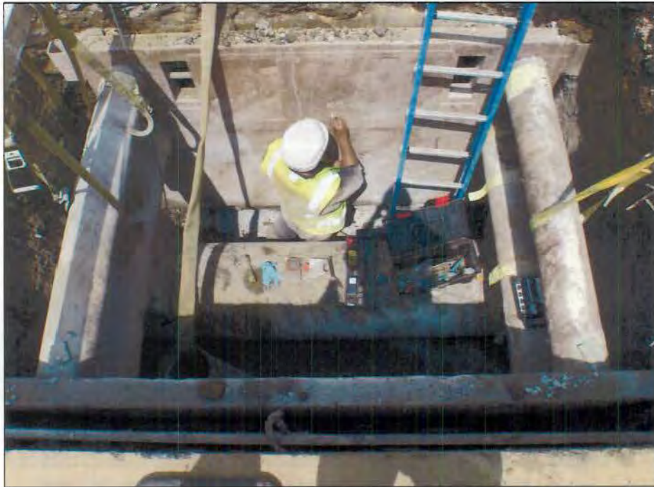
FIGURE A5.12 - PHOTOGRAPH OF PIPE IN EXCAVATION
