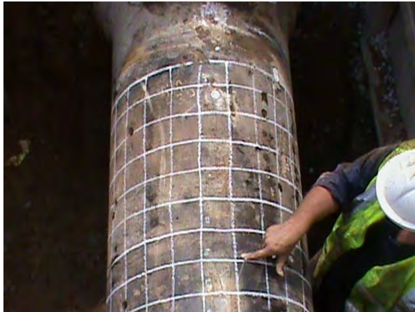
Figure 3-18. Grid Pattern Used for Ultrasonic Wall Thickness Measurements and Coating Assessment
