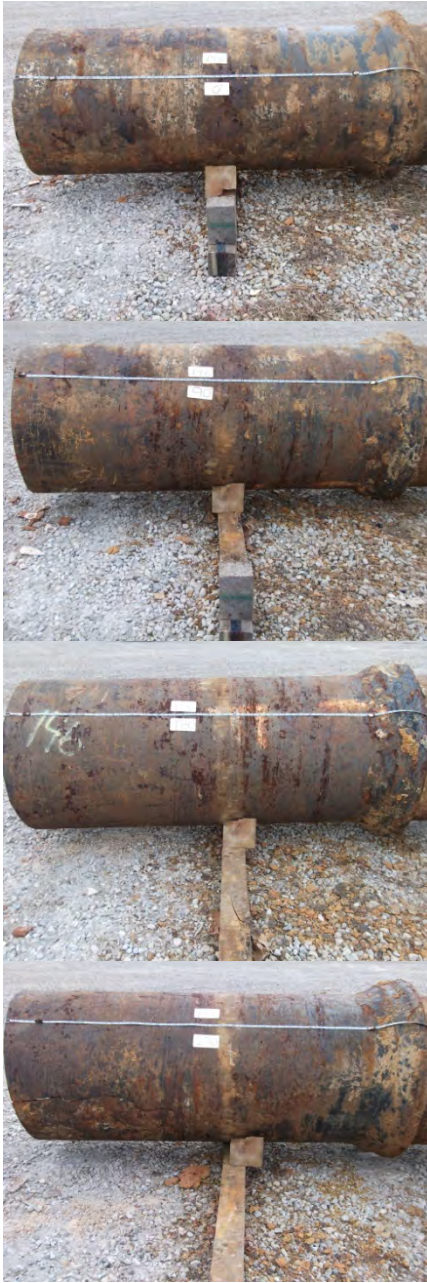
Figure A-146(1). Pipe 146 as Removed from Site
