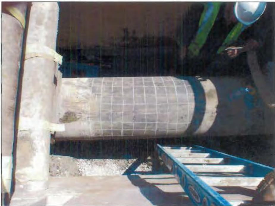
FIGURE A5.13 - PHOTOGRAPH OF COATING / CORROSION GRID
