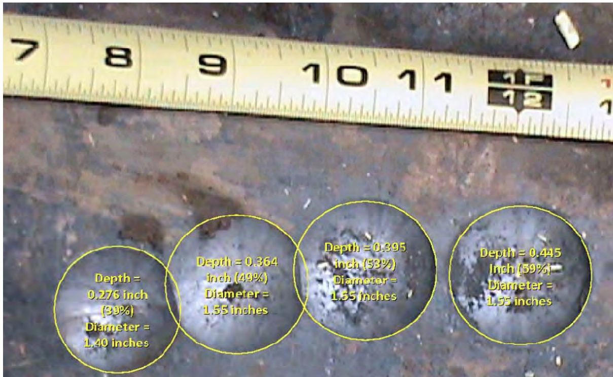
Figure 5-11. Calibration Defects in Pit F
