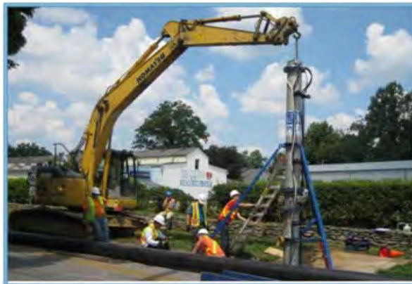
Setting up the PipeDiver extraction tube.
