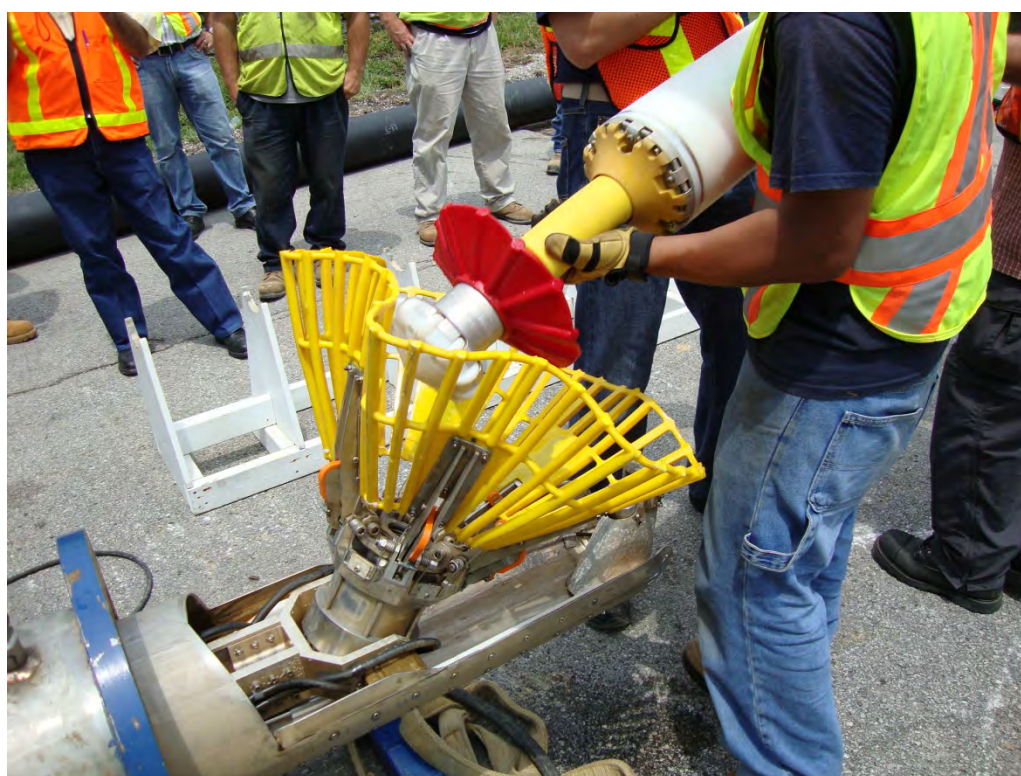
Figure 3-13. PipeDiver® Extraction Tube and Robotic Claw
