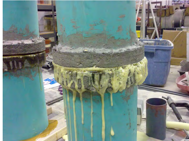
(b) Repaired cracked concrete with grout.
