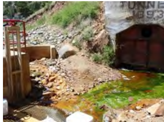
Figure 3. Argo Tunnel on right, sump region in lower left, and Big Five Tunnel and Virginia Canyon discharges in background left. Photo by Arcadis.
