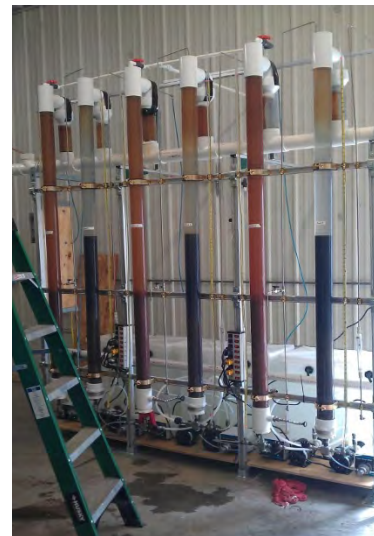
Figure 3. Pilot biological water treatment system for ammonia removal at the Palo, Iowa study site.
