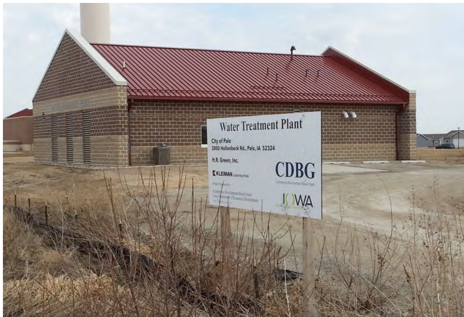
Figure 9. Water treatment plant building.
