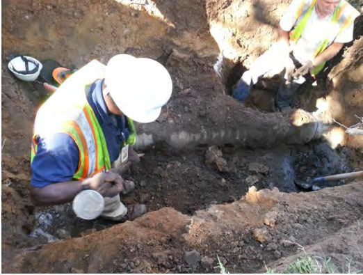
Figure B-52. Nashville 1: Retrieval of the Sample (left) and Measuring Annular Gap on the Received Sample (right)
