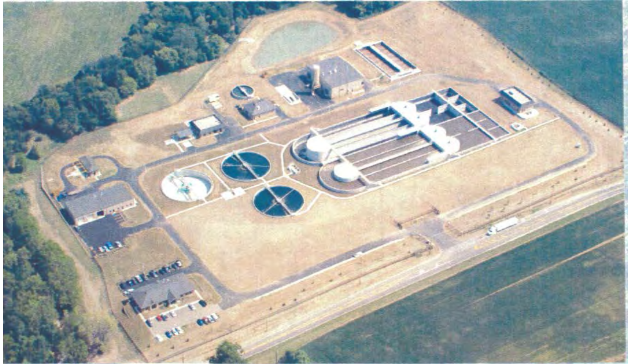
Figure 2.2. Aerial Photograph of Mason Water Reclamation Plant
