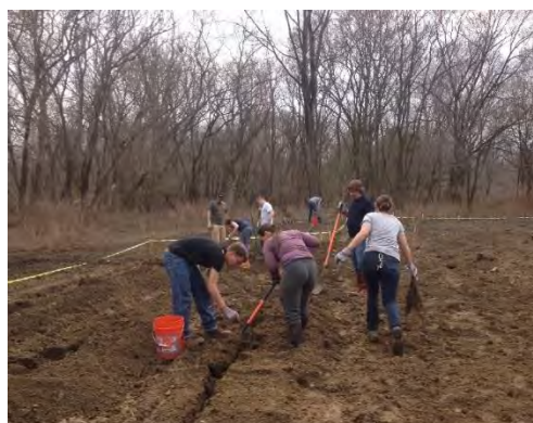
Figure 10. Tree and shrub planting for the evapotranspiration cap.
