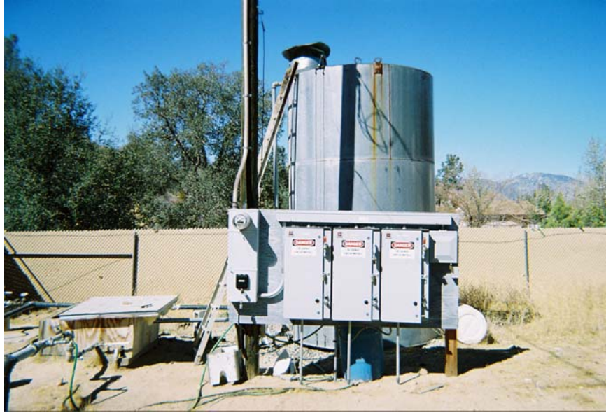
Figure 4-2. Preexisting Aeration Tank at Upper Bodfish in Lake Isabella, CA
