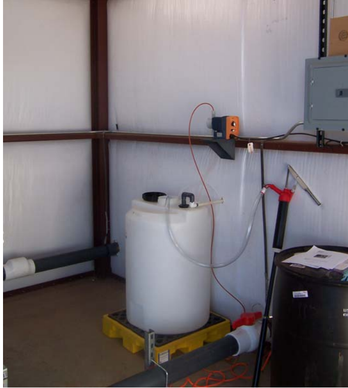
Figure 4-5. pH Adjustment System
