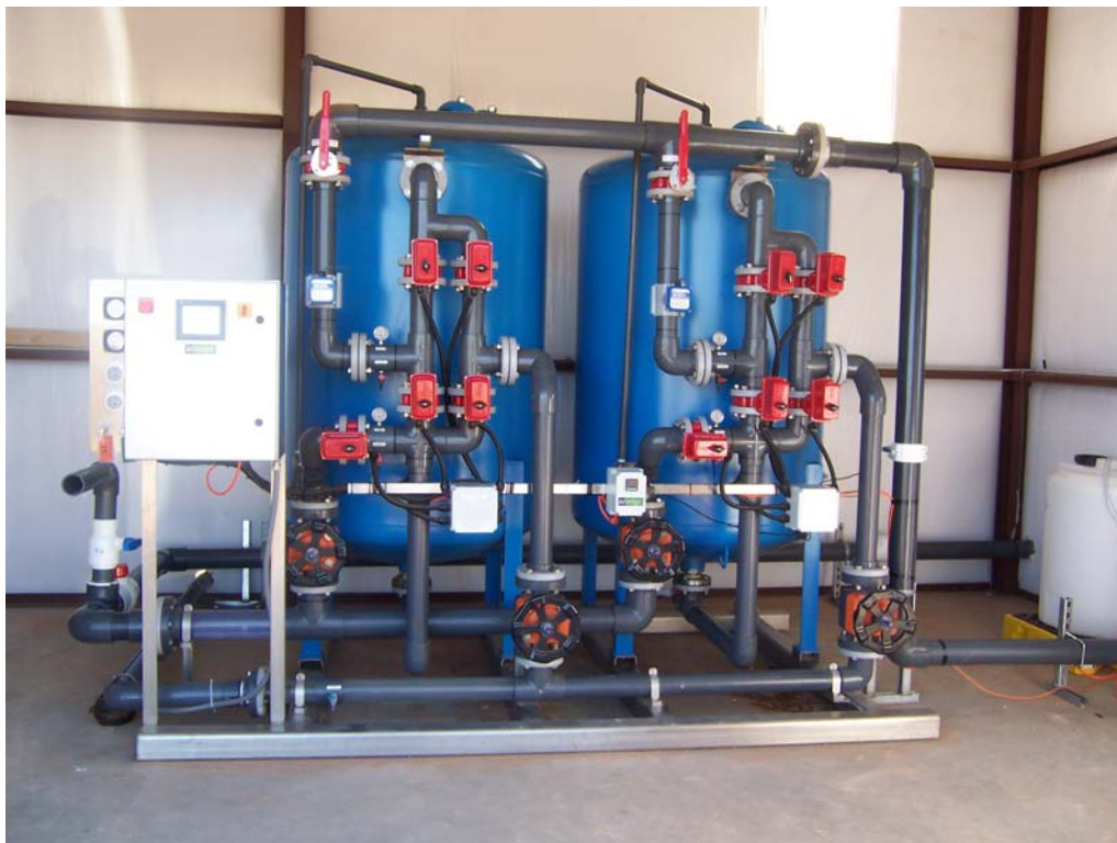
Figure 4-6. Adsorption System Valve Tree and Piping Configuration
