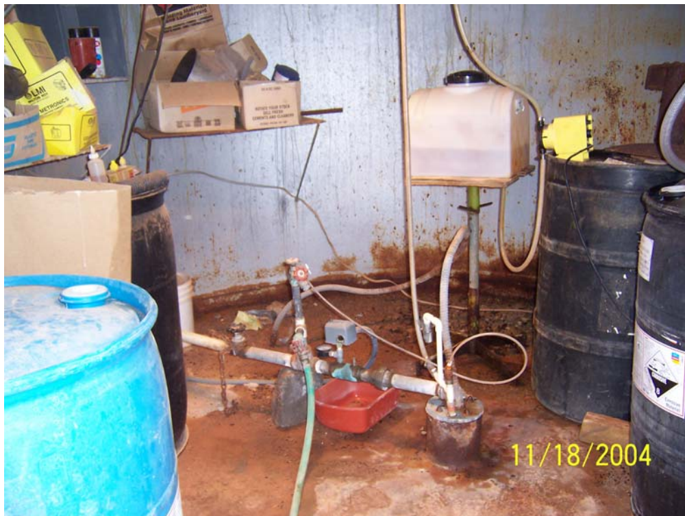
Figure 4-3. Pre-Existing Chlorine Addition System
