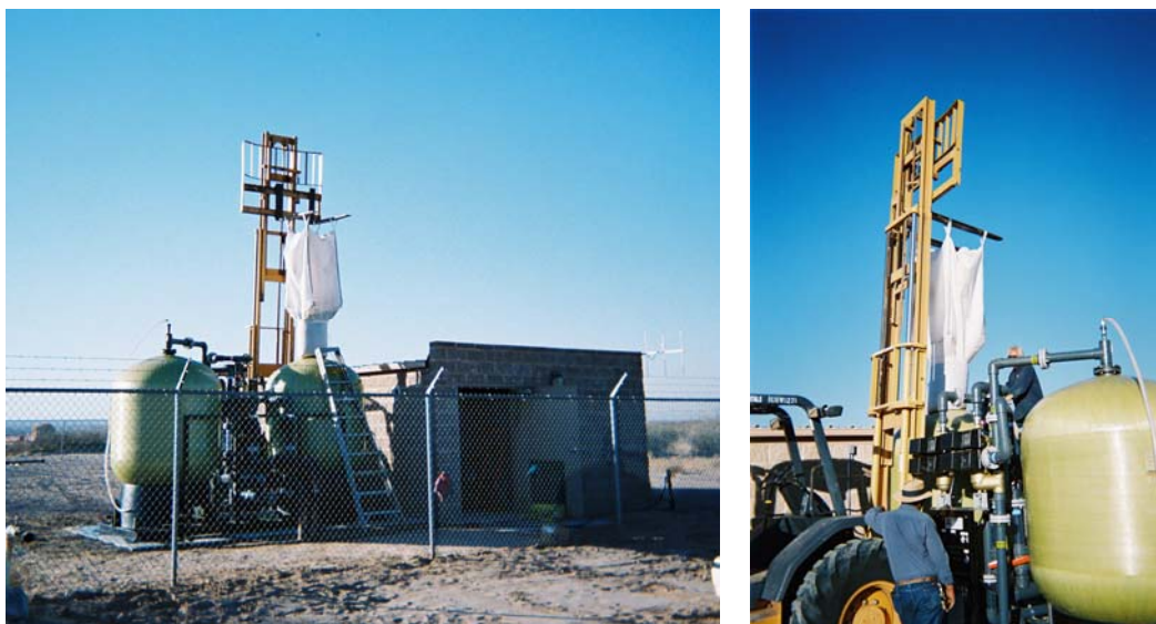
Figure 4-11. Media Loading to Adsorption Vessels
