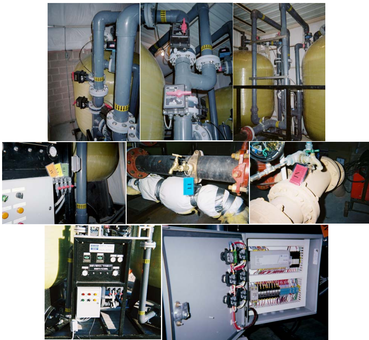
Figure 4-6. Treatment Process Components ( APU-300 System Valve Tree [top left and middle]; Backside of System Piping including Vessel Flow Meter Sensors [top right]; Sampling ports [middle]; and Control Panel [bottom])
