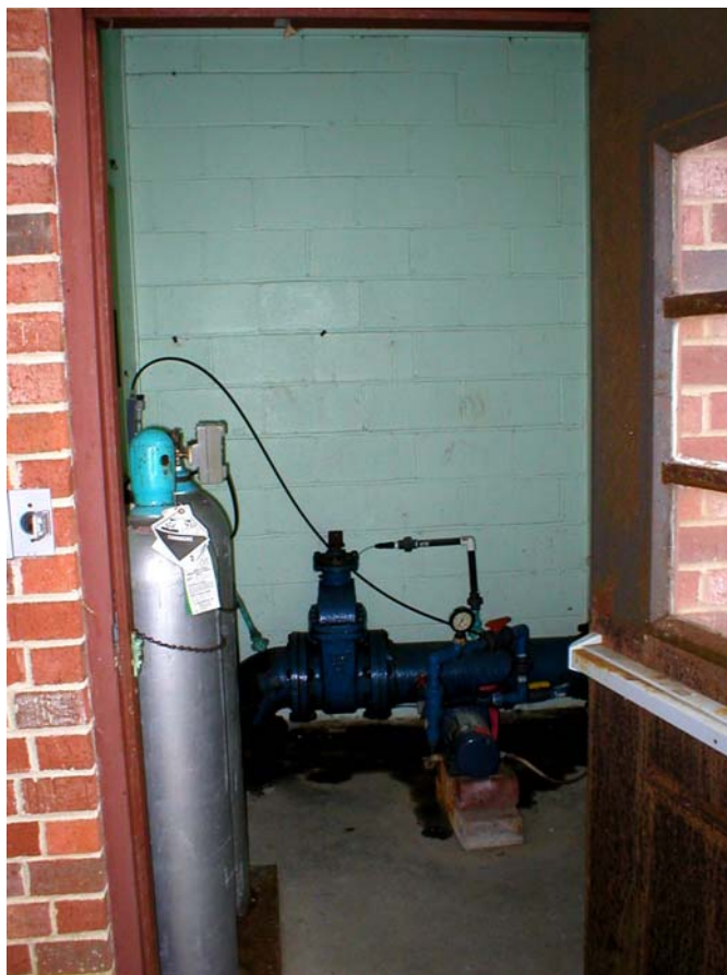
Figure 4-2. Chlorine Gas System at Well No. 1
