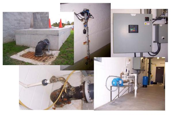
**Figure 4-5. Recycle System Components, Control, and Instrumentation** (Clockwise from Left: Concrete Recycle Tank and Overflow Piping; Float Switches; Recycle System Controller; Booster Pumps; and Recycle Water Injection Point)
