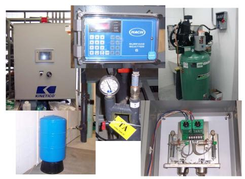
**Figure 4-4. Control and Instrumentation** (Clockwise from Left: Control Panel Housing PLC; Turbidimeter Display; Compressor; Sample Tap and Pressure Gauge; Pressure Tank; and Mercury Switch)
