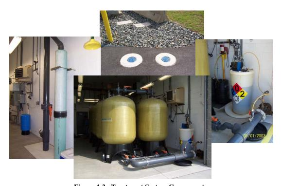
**Figure 4-3. Treatment System Components** (Clockwise from Top: Well No. 4 Bypass Valve; Well No. 4 Inlet with Iron Addition Point; Two Contact Tanks and Three Filtration Vessels; and Backwash Discharge Piping to Recycle Tank)
