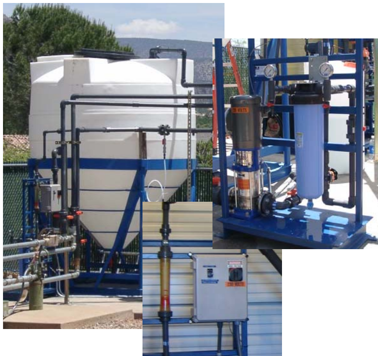
Figure 4-6. Backwash Process Components (Clockwise from Left: 1,800-gal Holding Tank; Recycle Pump and Bag Filter; and Backwash Flowrate Indicator and Pump Box)
