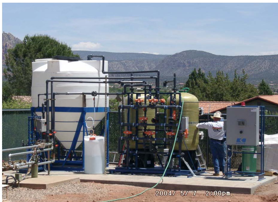
Figure 4-4. Kinetico's FA-236-AS Treatment System on Concrete Pad
