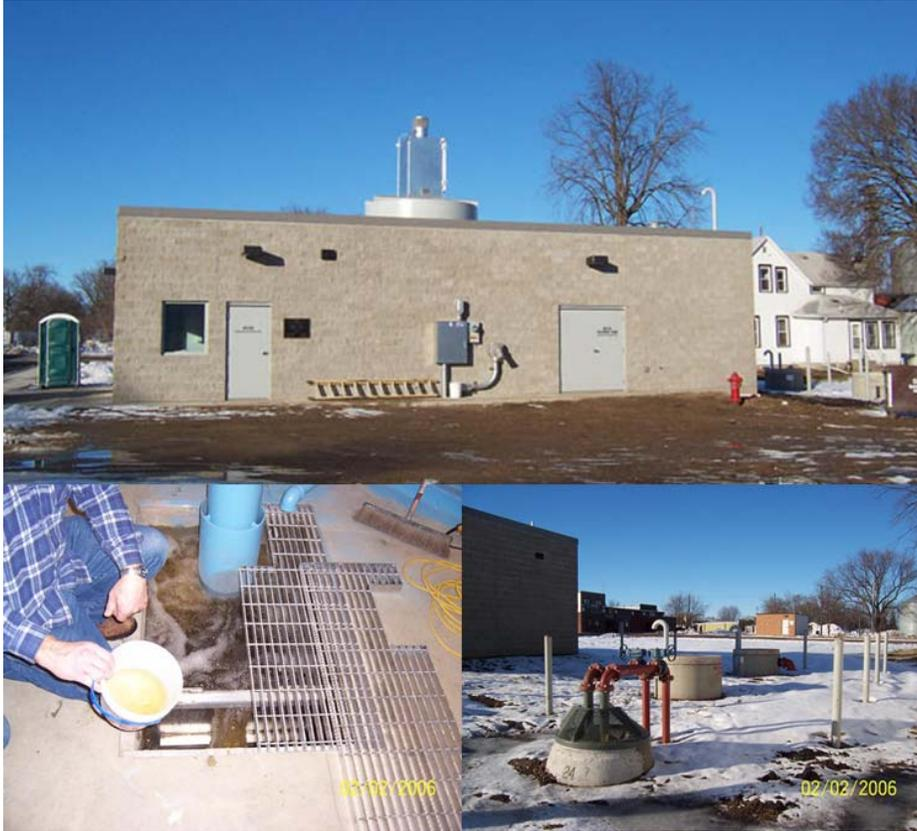
**Figure 4-10. Building with AERALATER® Tower (top), Backwash Sump (bottom left), and Backwash Water Holding Tanks (bottom right) at Stewart, MN**
