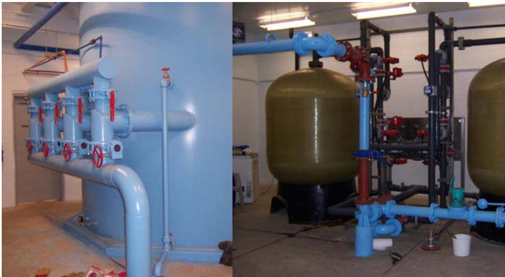
Figure 4-7. AERALATER® (left) and APU-300 Systems (right) at Stewart, MN
