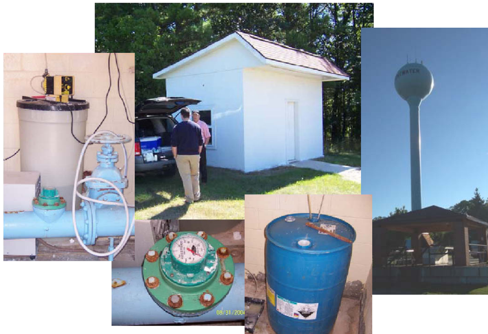
Figure 4-1. Existing Facility and System Components (Clockwise from Top: Well No. 2 Pump House, Water Tower, Polyphosphate Drum, Wellhead Totalizer, and Piping and Chlorine Addition Equipment)
