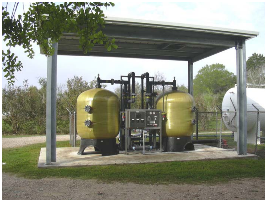
Figure 4-5. Photograph of APU-30S Arsenic Removal System
