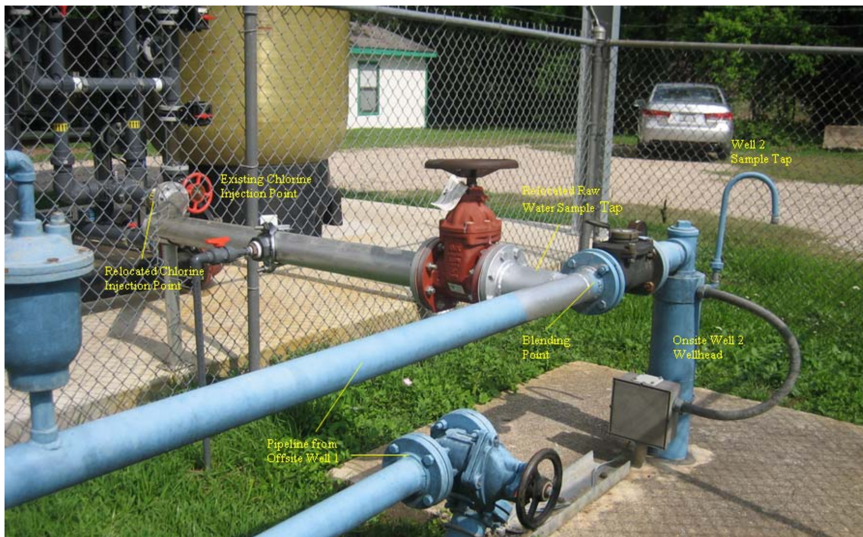
Figure 4-12. Photograph of Piping, Sample Taps, and Chlorine Injection Point Prior to Treatment System
