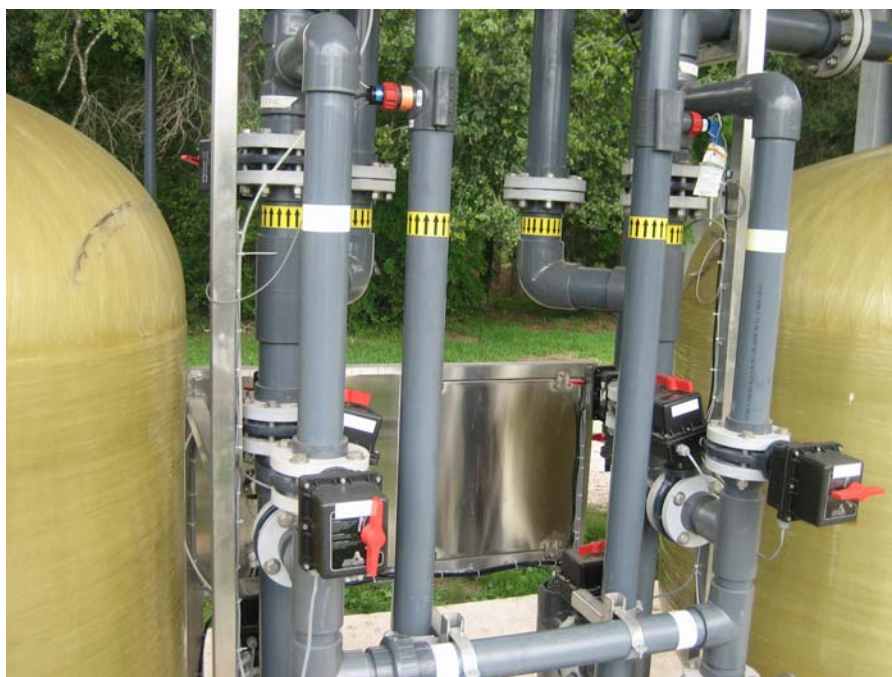
Figure 4-8. APU-30S System Valve Tree and Piping Configuration
