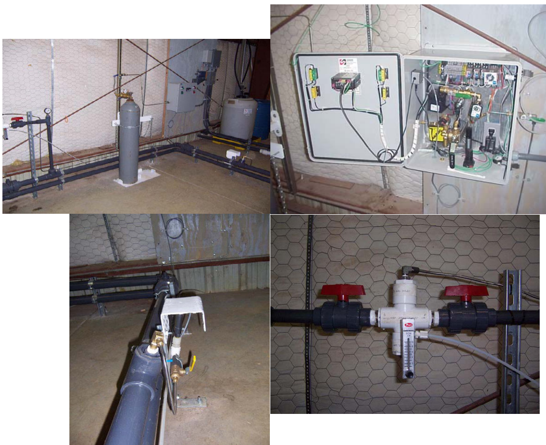
Figure 4-7. Carbon Dioxide Gas Flow Control System for pH Adjustment (Clockwise from Top Left: Liquid CO 2 Supply Assembly; Automatic pH Control Panel; CO 2 Membrane Module; Port for pH Probe)
