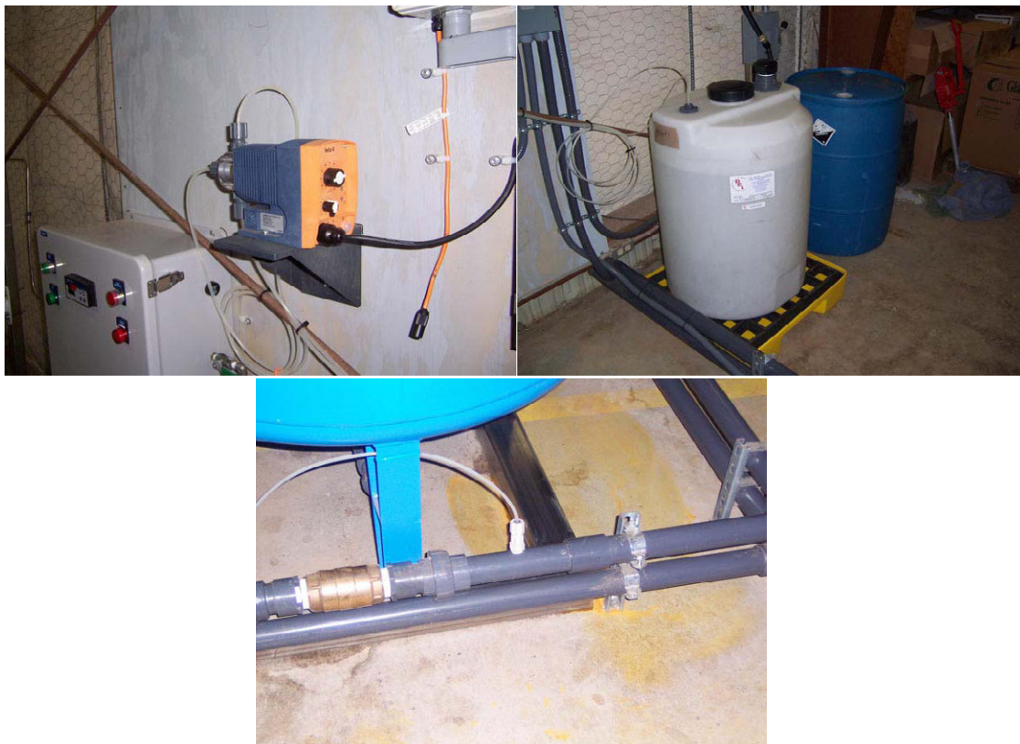
Figure 4-8. Chlorination Feed System (Clockwise from Top Left: Chlorine Metering Pump; HDPE Chemical Feed Tank with Secondary Containment; Chlorine Injection Port)
