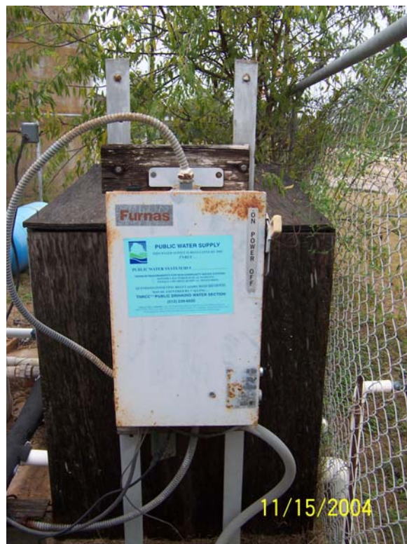
Figure 4-3. Existing Chlorine Addition System
