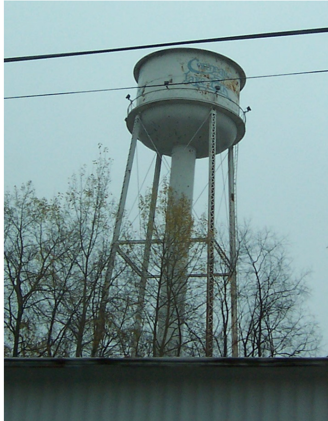
Figure 4-4. 75,000-gal Water Tower at Conneaut Lake Park
