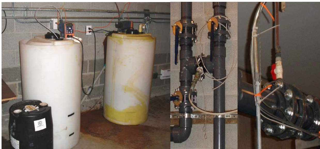
Figure 4-6. NaOCl and FeCl 3 Addition Systems (NaOCl day tank and pump [left-left side], FeCl 3 day tank and pump [left-right side], NaOCl injection point [center], and FeCl 3 injection point [right])
