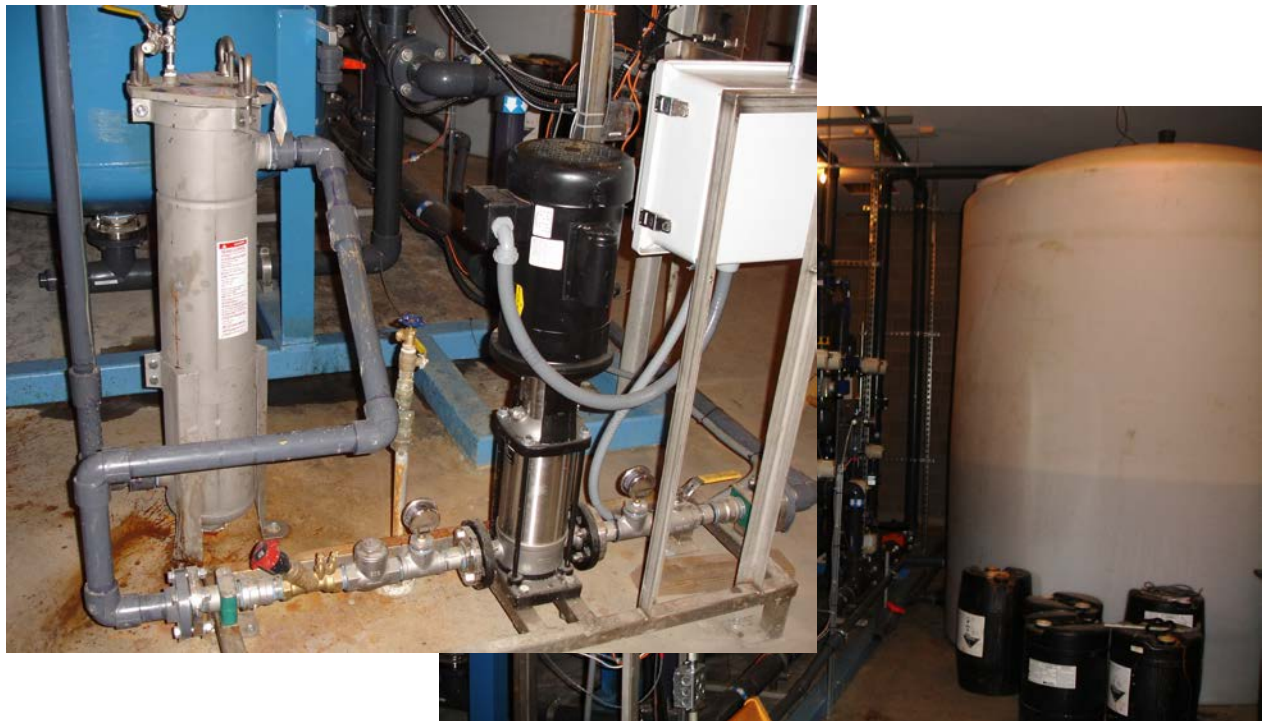
Figure 4-10. Backwash Reclaim System (Photograph on left: Bag Filter [left], Reclaim Pump [center], and Control Box [right]) (Photograph on right: Backwash Holding Tank)
