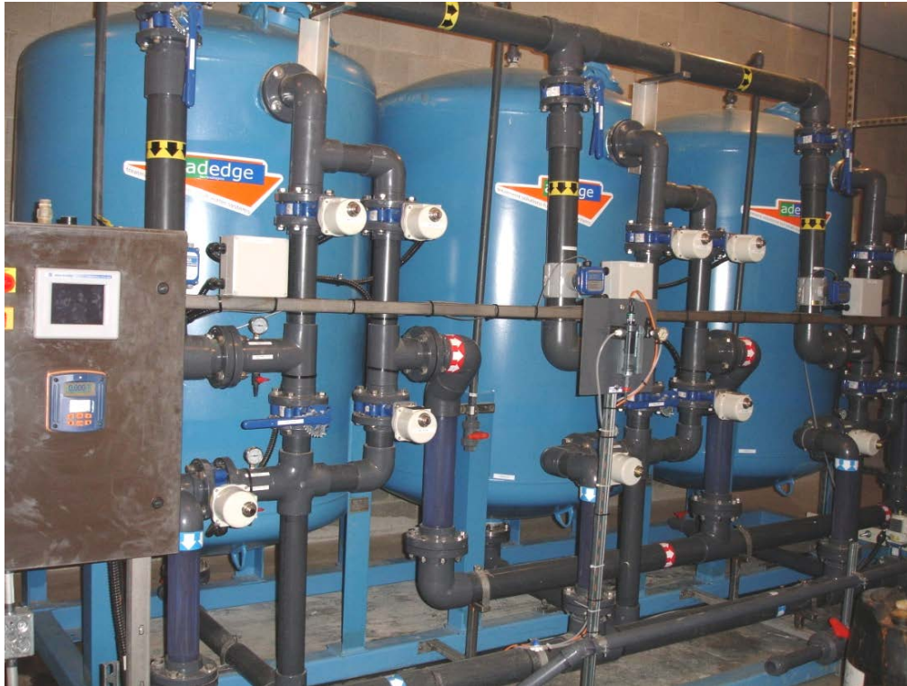
Figure 4-8. Carbon-Steel Filtration Vessels with Associated Piping and Valves
