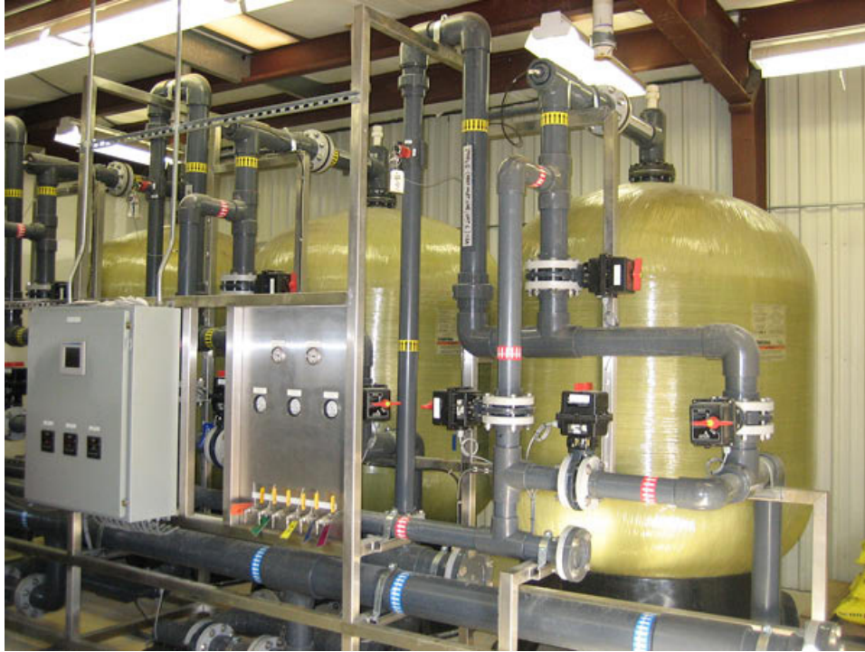
Figure 4-8. Photograph of APU-450 Arsenic Removal System
