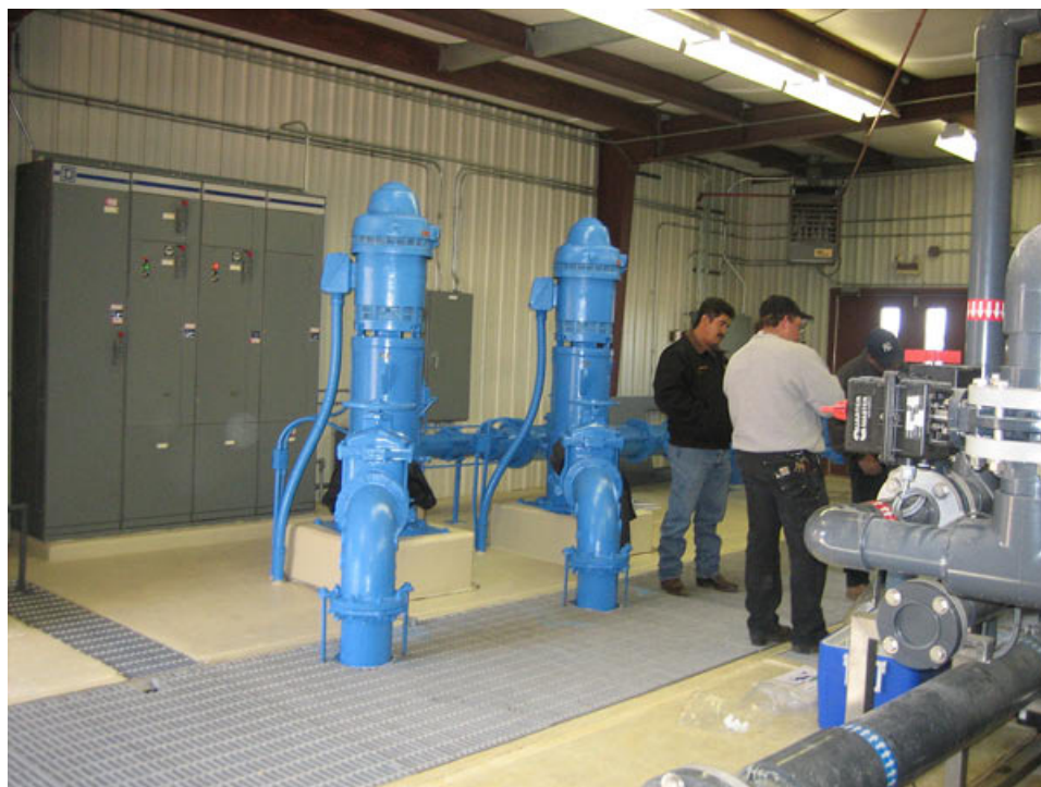
Figure 4-14. Modified Booster Pump Station
