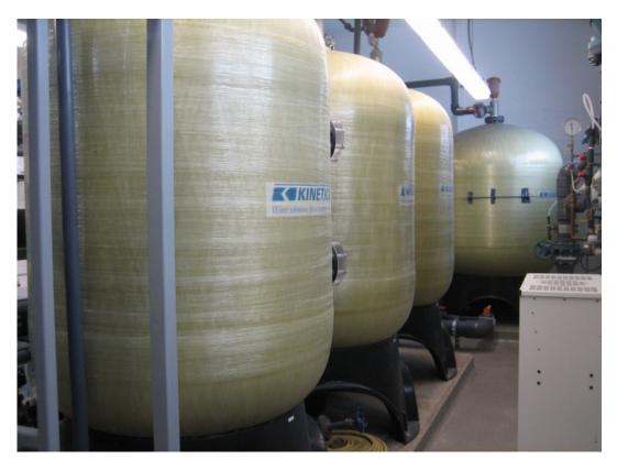
Figure 1. Three Macrolite<sup>®</sup> Filters (forground) and One Contact Tank (background)
