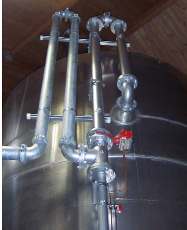
Figure 4-9. Blower Piping Modification
