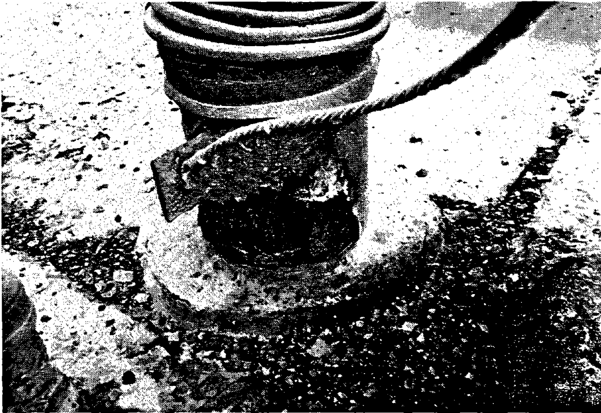
Figure 6-4. Example of rapper boot corrosion.
