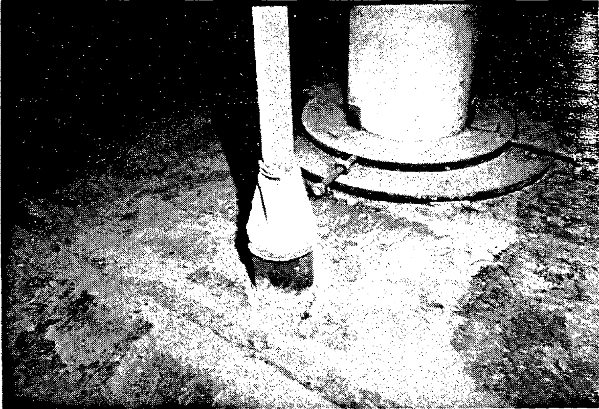
Figure 6-28. Jack screws.
