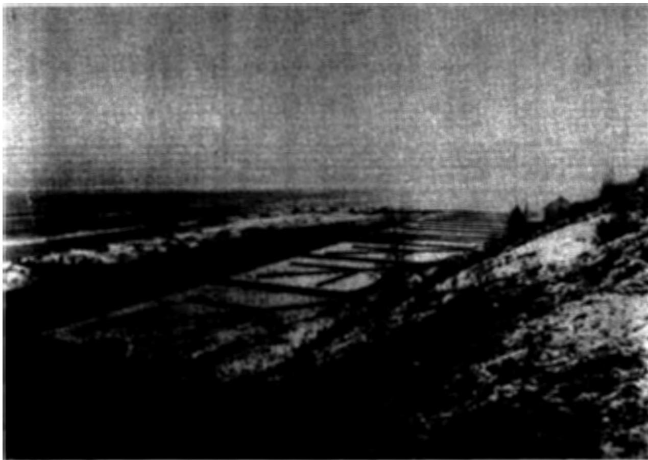
Figure 1. Village of Lake Forest's Intermittent Sand Filters, Year 1901
