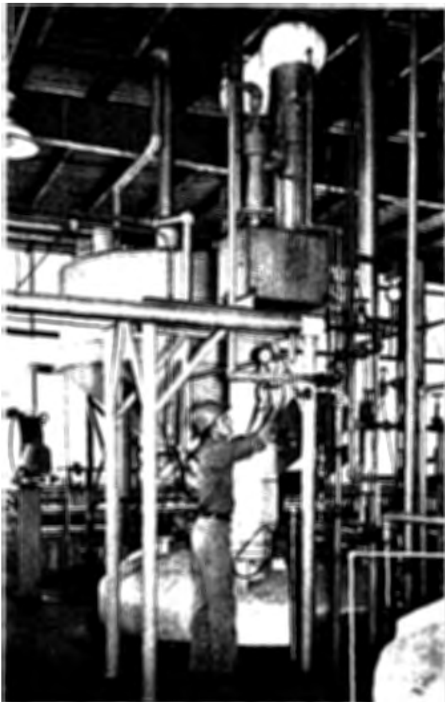
Figure 511. Venturi scrubber venting resin-manufacturing equipment (Silmar Chemical Corporation, Hawthorne, Calif.).
