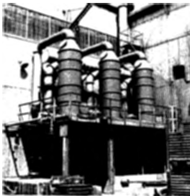
Figure 199. High-efficiency packed-column water scrubbers used with a baghouse for control of emissions from chlorine fluxing and dross processing.
