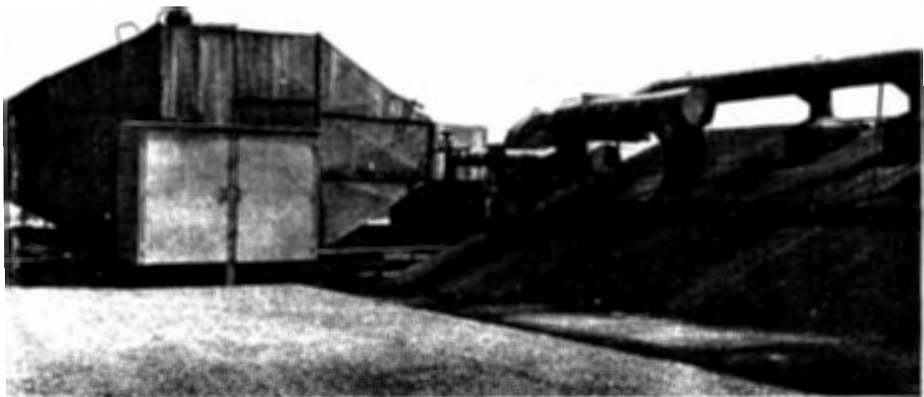
Figure 549. A two-stage precipitator and wet centrifugal collector venting smokehouses (The Rath Packing Co., Vernon, Calif.).
