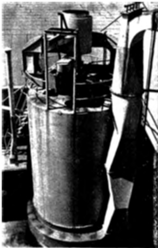
Figure 561. A chlorinator-scrubber odor control system venting a fish meal drier (Star-Kist Foods, Inc., Terminal Island, Calif.).
