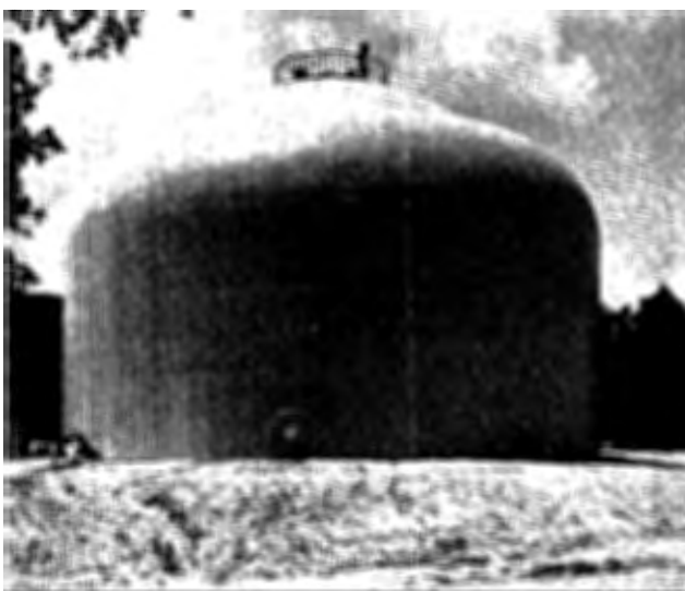
Figure 432. Types of pressure vessels: (upper left) 51-foot-diameter spheres (Bu-tane is stored in these spheres at a petroleum refinery in California. Capacity of each is 15,000 barrels, diameter is 54 feet 9 inches and design working pressure is 35 pounds per square inch.); (upper right) two 5,000-barrel spheroids designed for 20-psi pressure; (lower left) large noded spheroids, each designed for 100,000-barrel capacity and 15-psi pressure; (lower right) a 20,000-barrel noded hemispheroid designed for 2-1/2-psi pressure (Chicago Bridge and Iron Company (1959).
