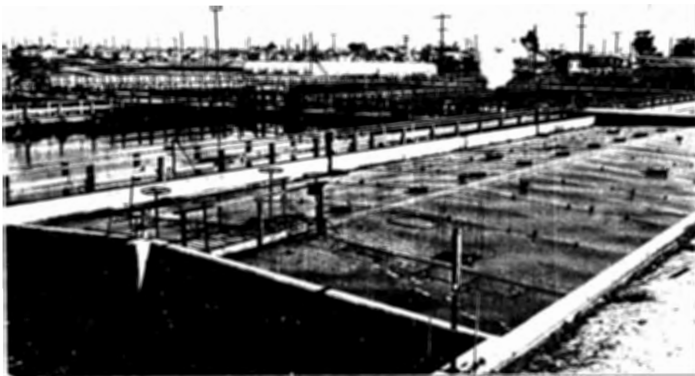
Figure 488. Floating-roof cover on refinery oil-water separator (Union Oil Company of California, Los Angeles, Calif.).
