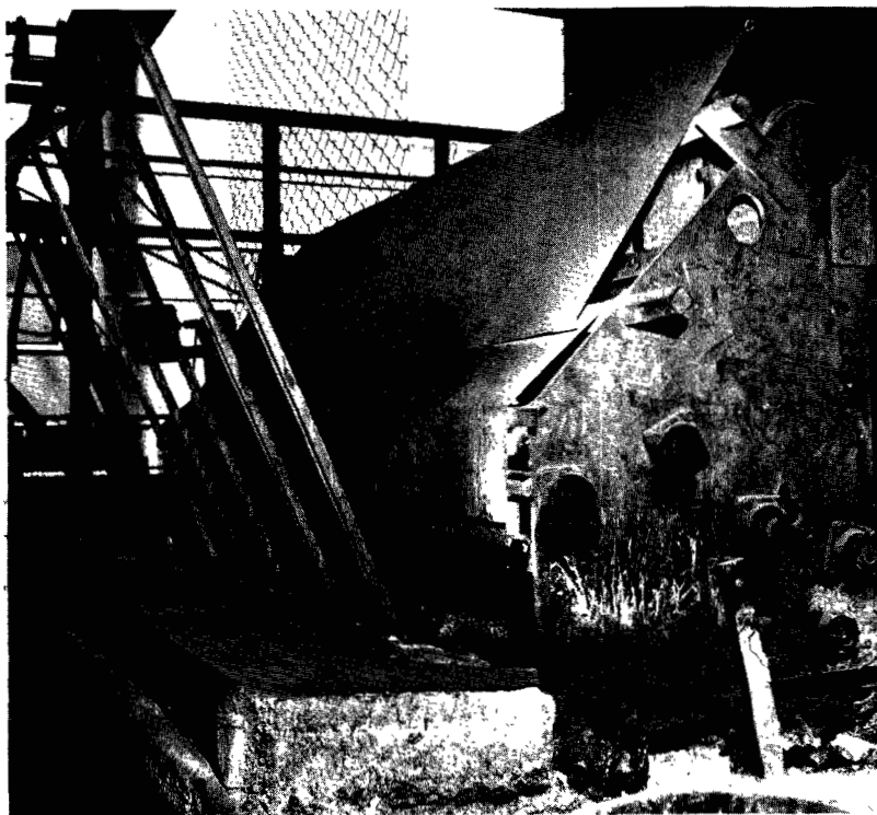
Figure 302. Slot-type hood serving a chain link fence-galvanizing flux box (Anchor Post Products, Inc., of California, Whittier, Calif.).
