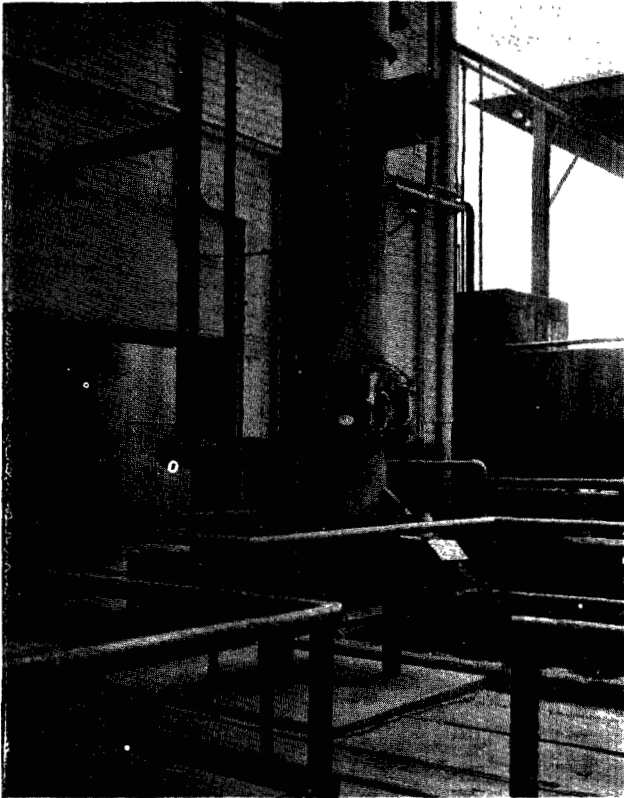
Figure 103. Direct-fired afterburner controlling odorous emissions from animal matter-rendering equipment (Peterson Manufacturing Co., Inc., Los Angeles, Calif.).
