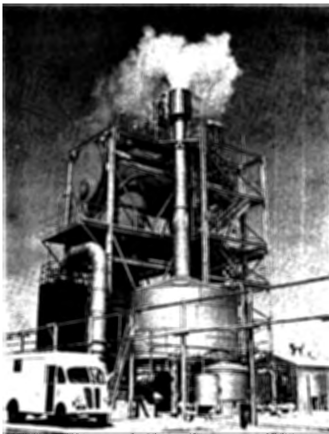
Figure 521. Phosphoric acid plant with a Raschig ring-packed scrubber.
