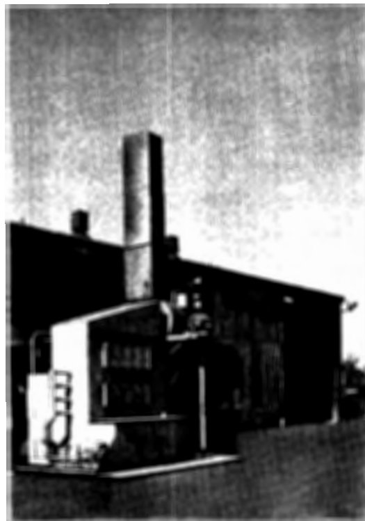
Figure 303. Water-wash scrubber serving a continuous chain link galvanizing kettle.
