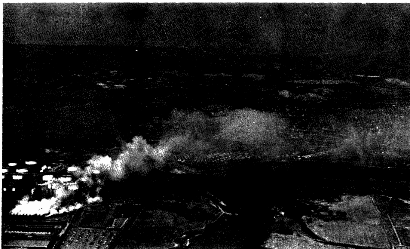
Figure 391. A fluid catalytic cracking unit as a source of a visible plume. Use of a carbon monoxide waste-heat boiler eliminates this plume formation.
