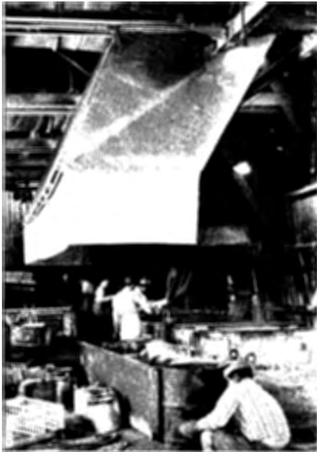
Figure 300. High-canopy hood over a galvanizing kettle (Superior Pacific Galvanizing Company, Inc., Los Angeles, Calif.).
