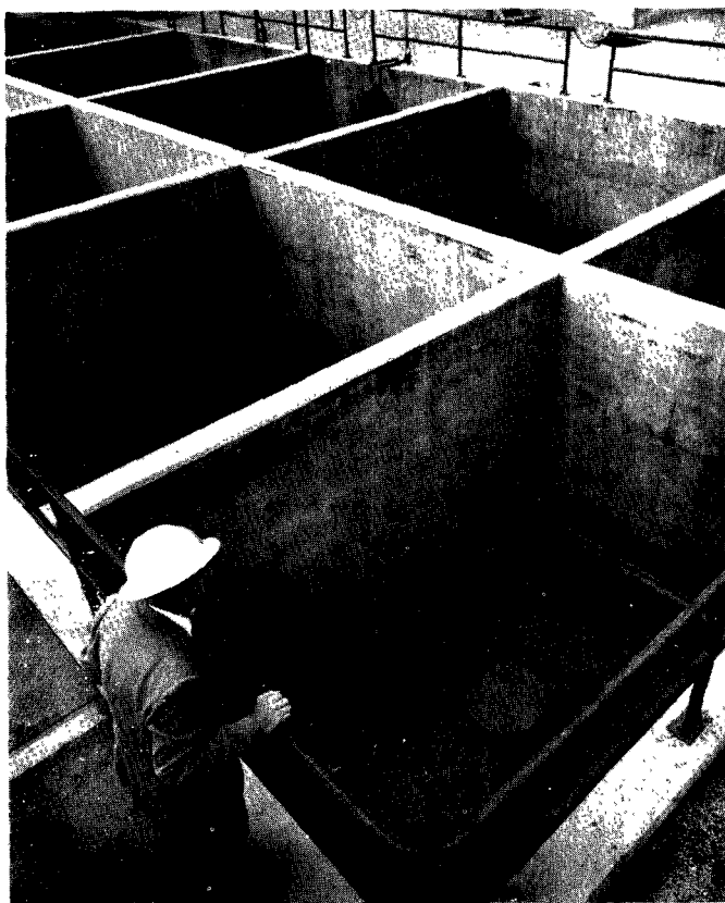
Figure 489. Floating roof on refinery oil-water separator (Atlantic-Richfield Oil Company, Los Angeles, Calif.).
