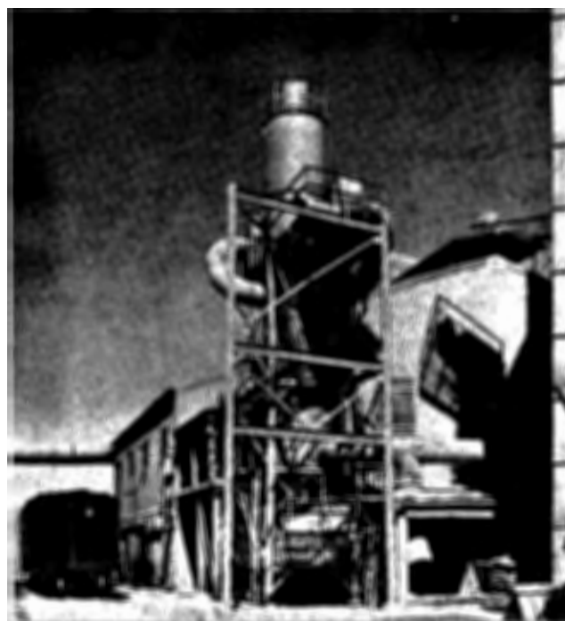
Figure 535. Wet, centrifugal-type scrubber controlling emissions from a glass-melting furnace (Thatcher Glass Co., Sangus, Calif.).
