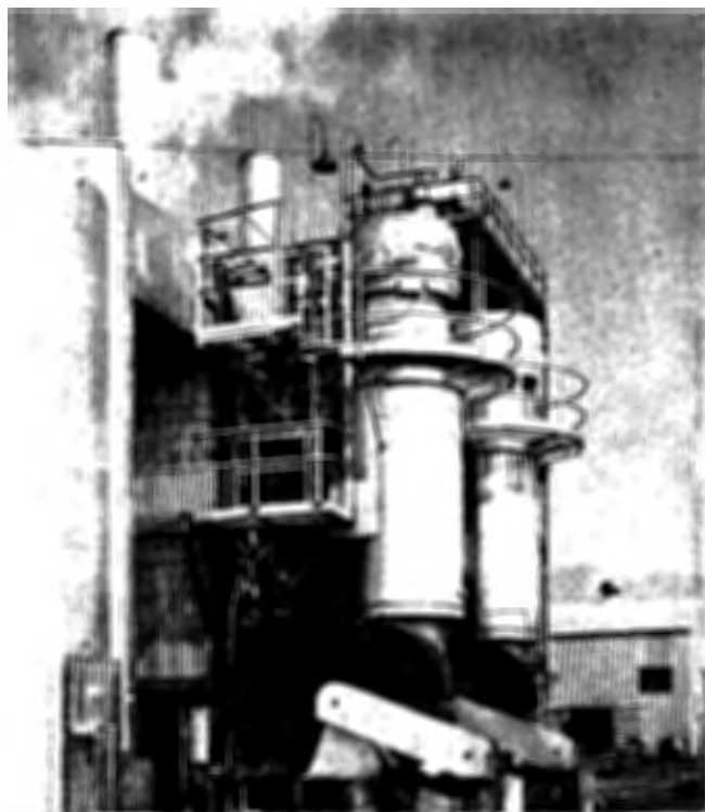
Figure 106. Emissions from two phthalic anhydride production units being controlled by direct-fired afterburners (Reichhold Chemicals, Inc., Azusa, Calif.).
