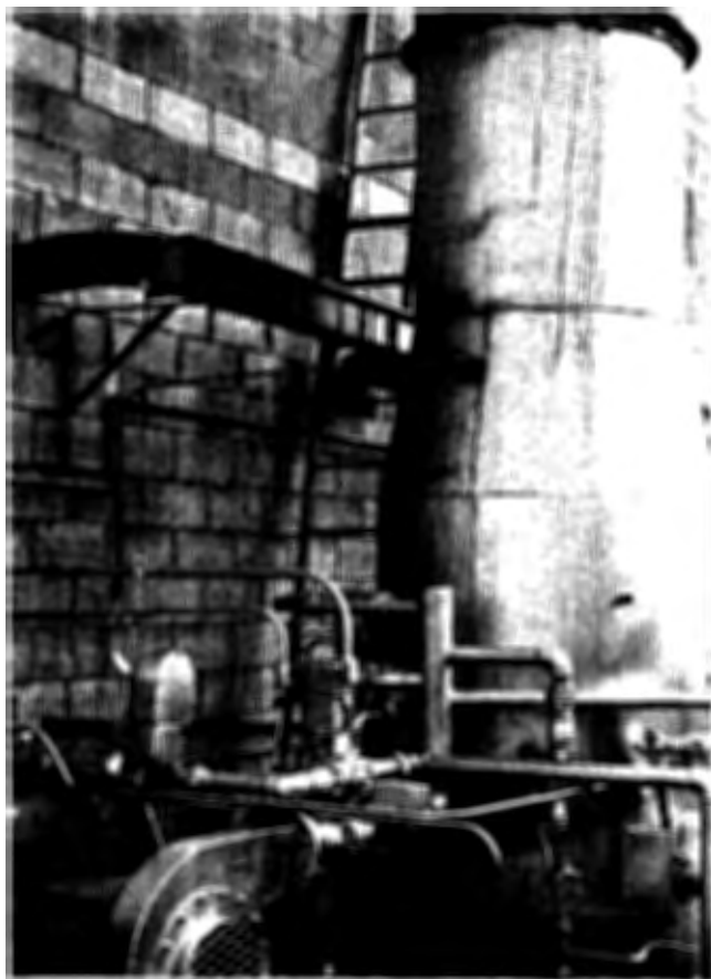
Figure 99. Direct-fired afterburner venting three varnish-cooking kettles (Standard Brand Paint Co., Torrance, Calif.).
