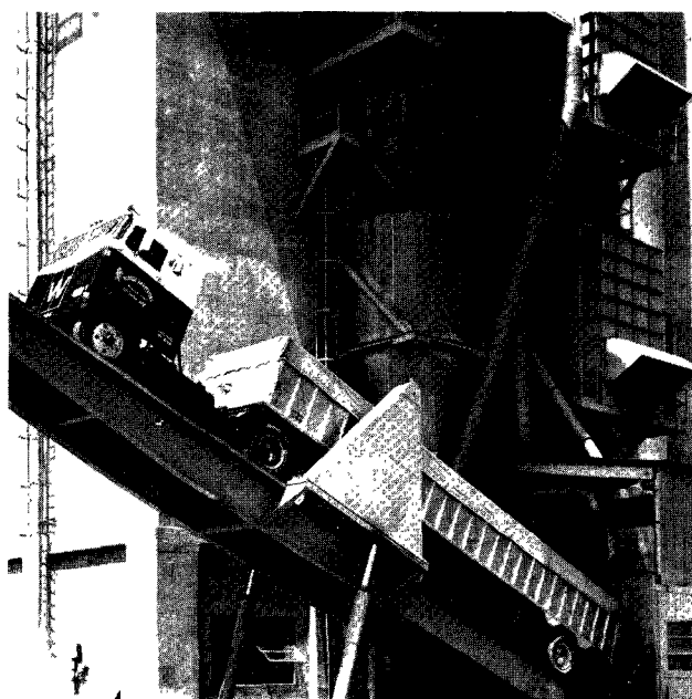
Figure 255. Truck-receiving station with baghouse control of the receiving hopper (Koppel Bulk Terminal, Long Beach, Calif.; and Wunsch Harvesters, Phoenix, Ariz.).
