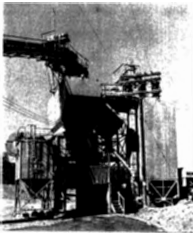
Figure 233. Overall view of wet- and dry-concrete-batching plant and baghouse located at a California Freeway project (Guy F. Atkinson Co., Long Beach, Calif.).
