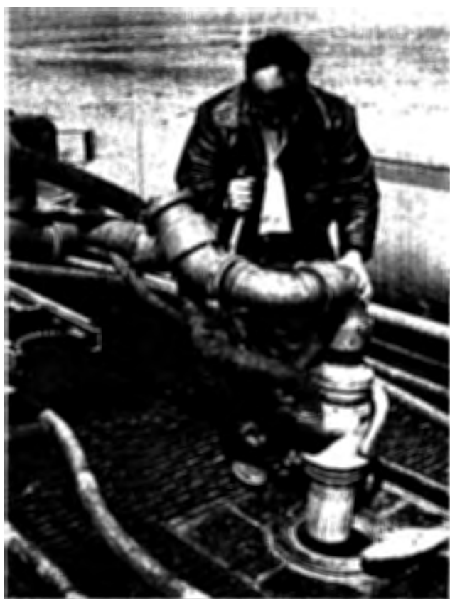
Figure 471. Closeup view of SOCO vapor closure, withdrawn position (American Airlines, Los Angeles, Calif.).
