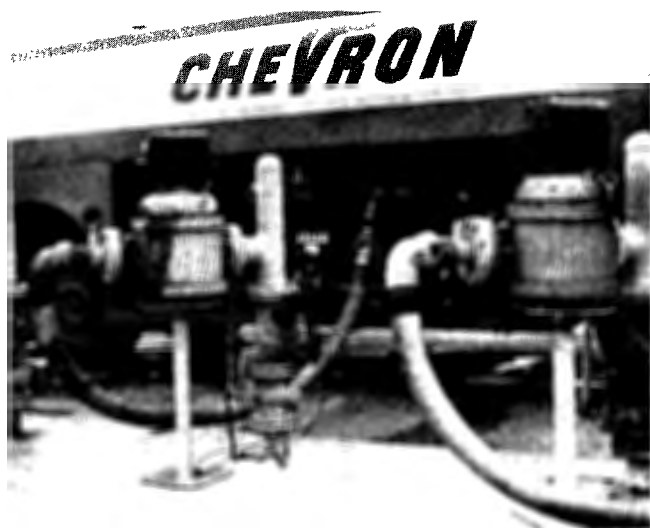
Figure 476. Bottom loading of tank trucks provides one way to collect vapor during loading in conjunction with the use of return line to storage tanks (Standard Oil Company of California, Western Operations, Inc., Los Angeles, Calif.).
