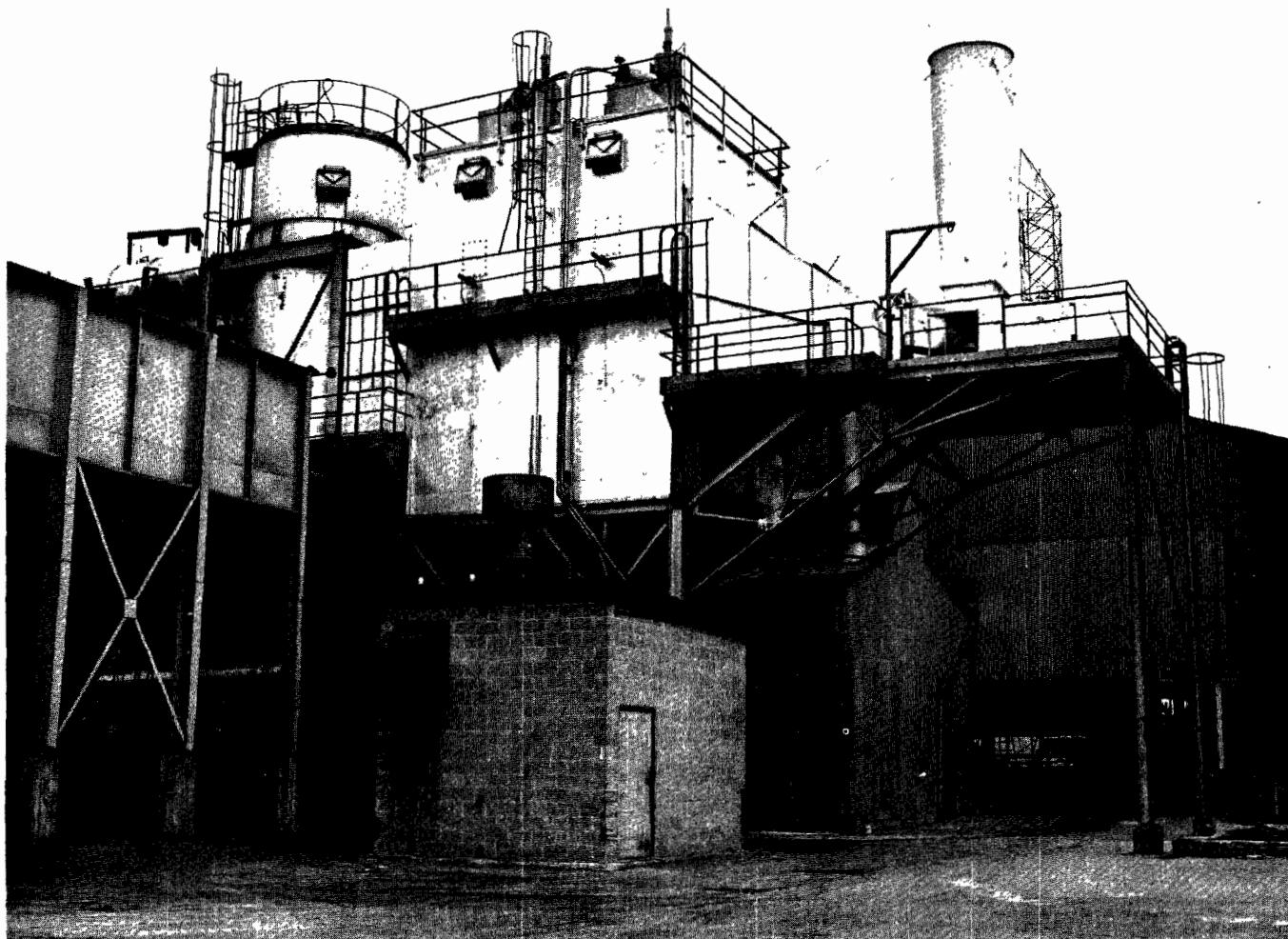
Figure 181. Photograph of an electrical precipitator preceded by a water spray conditioning chamber, vented cupola and afterburner not shown (Alabama Pipe Company, Southgate, Calif.).
