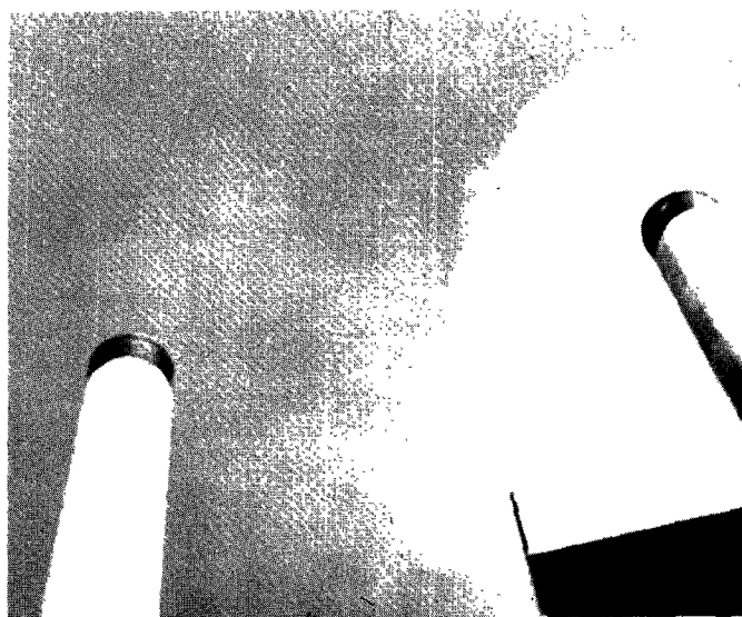
Figure 413. Exhaust gases from identical steam generators showing visible plume from oil-fired unit (right) as compared with clear stack of gas-fired unit (left).
