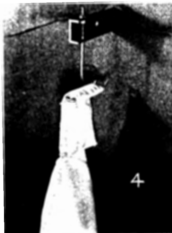
Figure 74. Method of hanging filter bags with strap top: (1) The end of the strap on the tube is brought up between the two horizontal bars of the tube hook. (2) The strap end is folded over the bar, directly under the vertical threaded spindle. (3) The remainder of the strap and the tube proper are brought up and over to the left, with the strap wrapping around the offset horizontal bar of the tube hook, and lying on, or over, the other end of the strap, originally threaded through the hook. The bag, as shown, can be raised, if necessary, by pulling with the right hand on the other end of the strap. (4) The correctly installed tube. Note that the tube proper hangs directly under the vertical threaded spindle of the tube hook (Wheelabrator Corporation, Mishawaka, Ind.).
