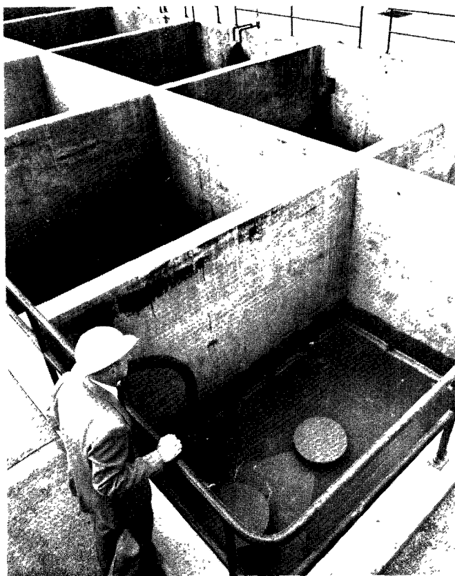
Figure 530. Floating roof on refinery oil-water separator (Atlantic-Richfield Oil Company, Los Angeles, Calif.).
