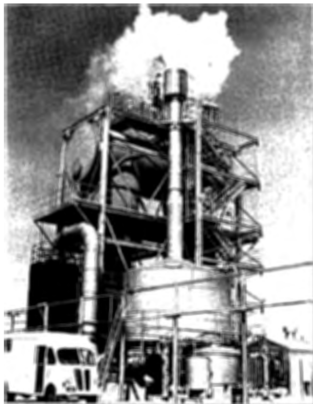
Figure 568. Phosphoric acid plant with a Raschig ring-packed scrubber.
