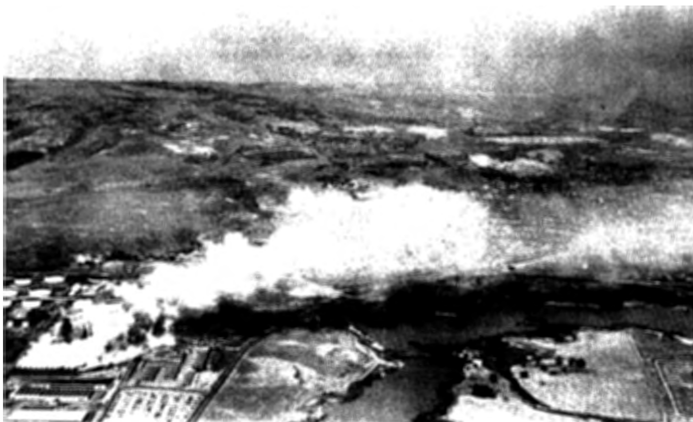
Figure 430. A fluid catalytic cracking unit as a source of a visible plume. Use of a carbon monoxide waste-heat boiler eliminates this plume formation.
