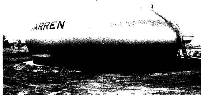
Figure 473. Types of pressure vessels: (upper left) 51-foot-diameter spheres (Butane is stored in these spheres at a petroleum refinery in California. Capacity of each is 15,000 barrels, diameter is 54 feet 9 inches and design working pressure is 35 pounds per square inch.), (upper right) two 5,000-barrel spheroids designed for 20-psi pressure; (lower left) large noded spheroids, each designed for 100,000-barrel capacity and 15-psi pressure; (lower right) a 20,000-barrel noded hemispheroid designed for 2-1/2-psi pressure (Chicago Bridge and Iron Company (1959).
