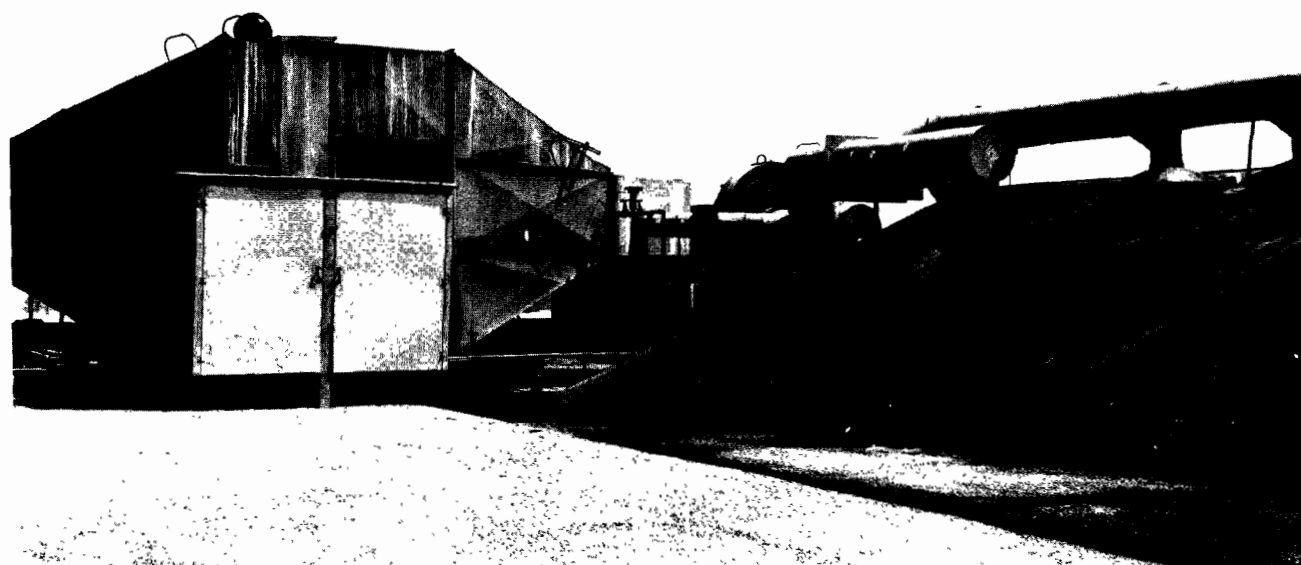
Figure 609. A two-stage precipitator and wet centrifugal collector venting smokehouses (The Rath Packing Co., Vernon, Calif.).
