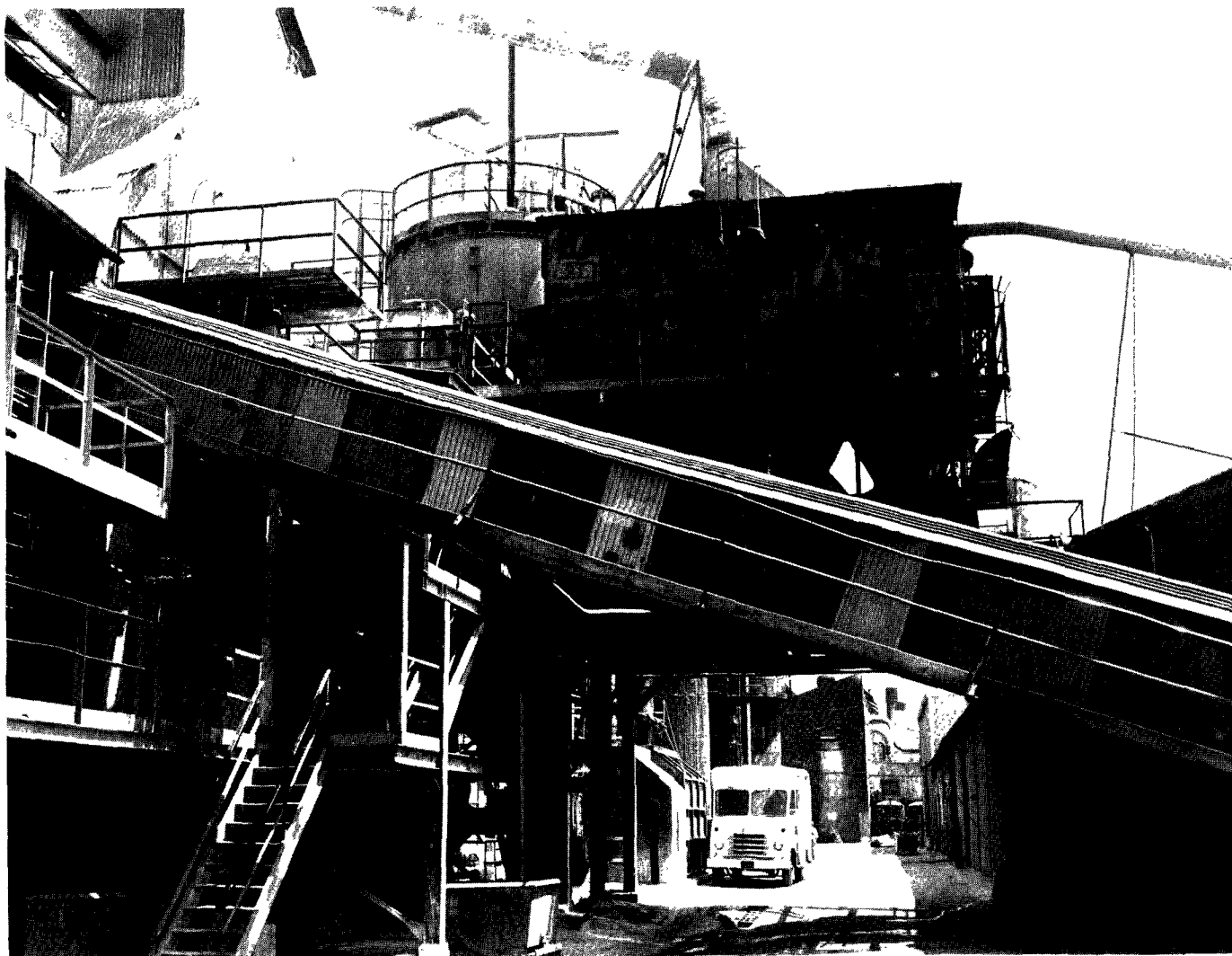
Figure 284. Baghouse venting sand applicator and belt conveyor for mineral dust (The Flintkote Co., Los Angeles, Calif.).
