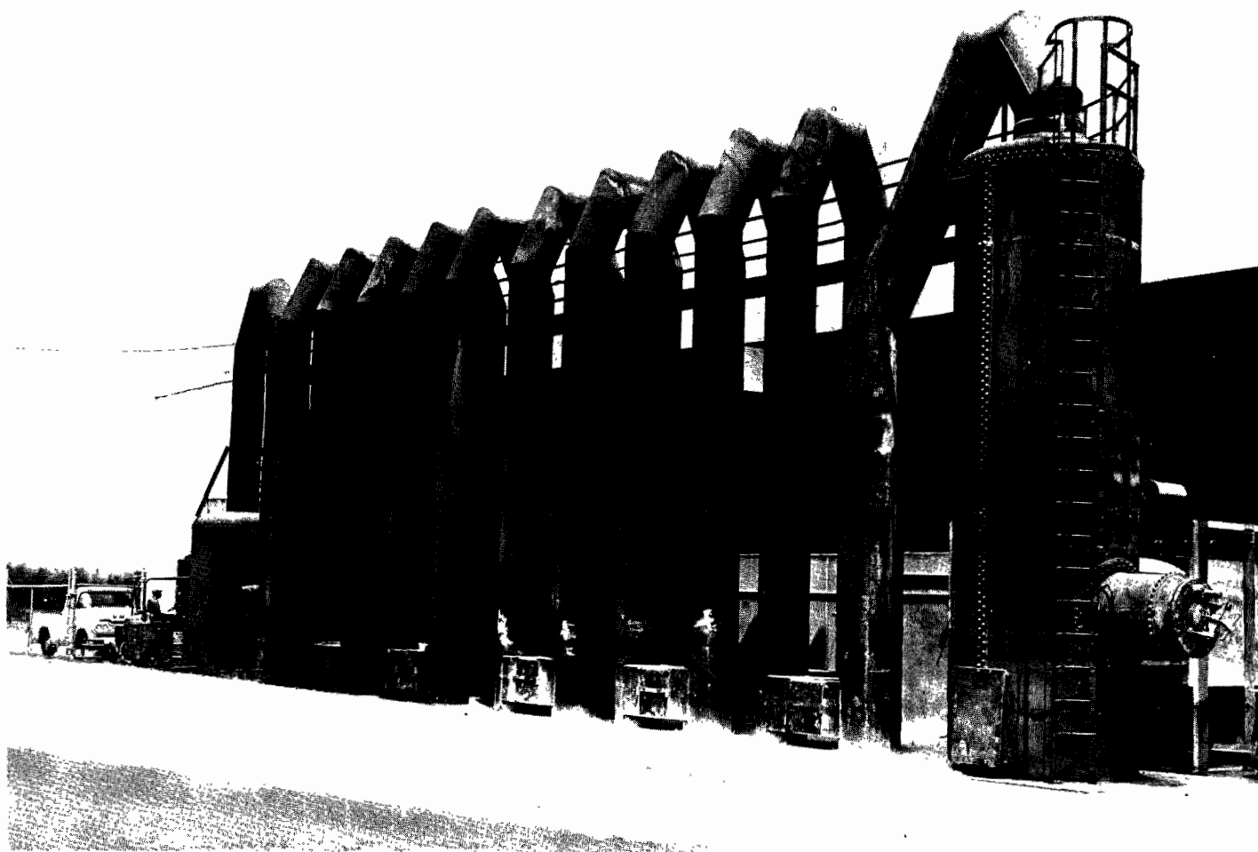
Figure 42. Radiation-convection cooling columns in an air pollution system serving a lead blast furnace and a lead reverberatory furnace (Western Lead Products Company, City of Industry, California).
