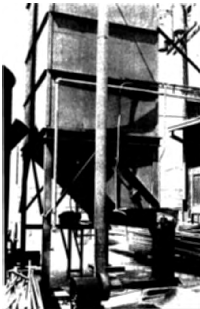
Figure 354. Feed bin with sloping bottom (California Moulding and Trim Mfg. Co., Los Angeles Calif.).
