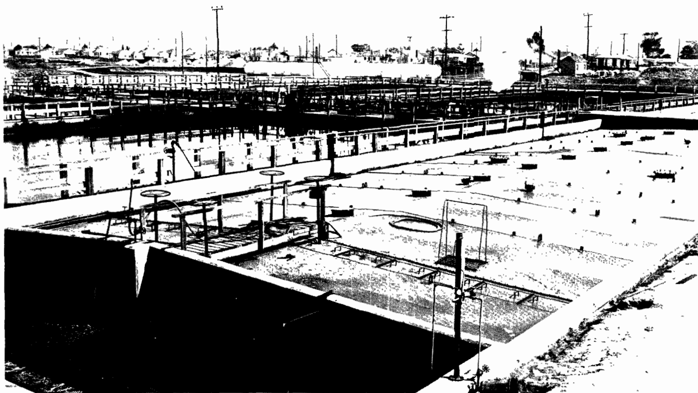
Figure 529. Floating-roof cover on refinery oil-water separator (Union Oil Company of California, Los Angeles, Calif.).
