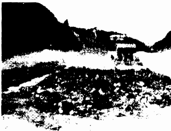
a. DOZER RIPPING LANDFILL LIFT COVER SOIL PRIOR TO SLUDGE APPLICATION.
