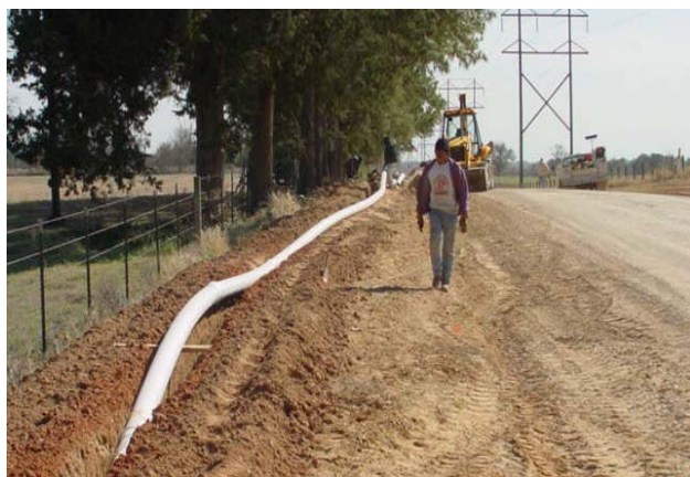
G&W laying new service lines and distribution mains
