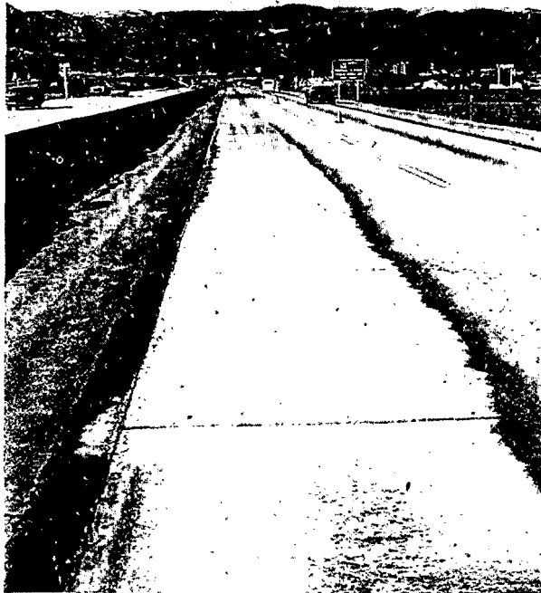
Figure 6-4 First One-Half Lane Strip of Formulation B Applied to Highway 36 Concrete
