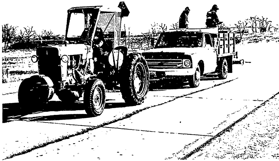
Figure 6-2 Entire Application Rig During Coating of Highway 36
