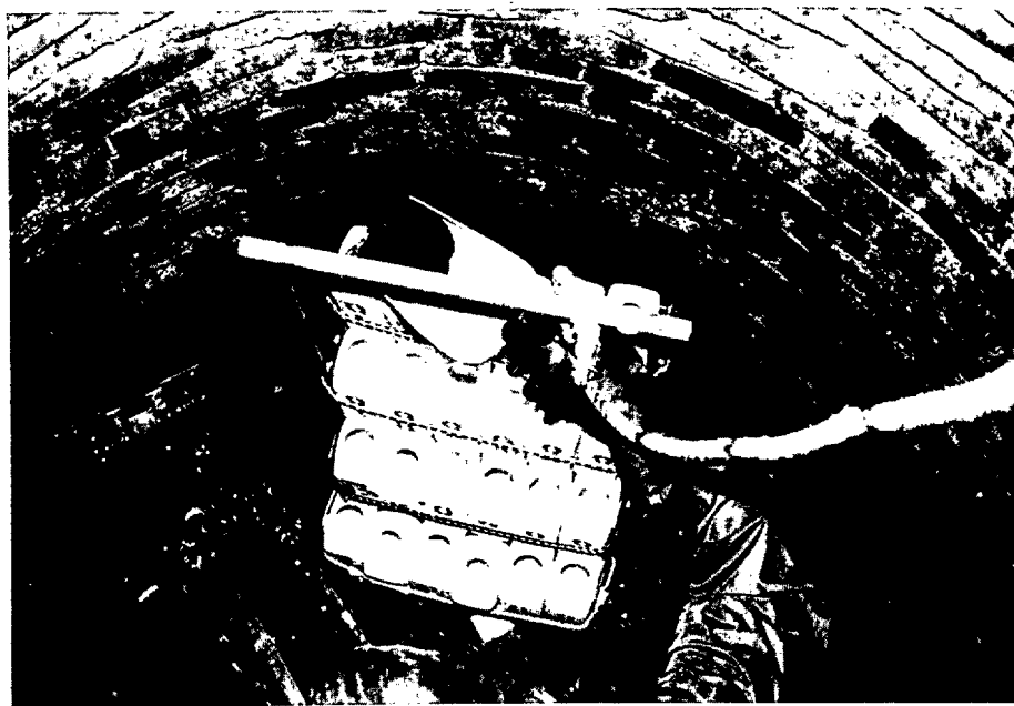
FIGURE 16: PHOTOGRAPHS OF SEDIMENT SCRAPING OPERATION
