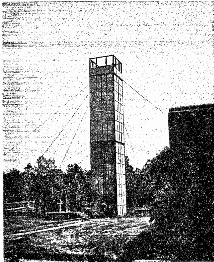
Figure 8. Dowpac HCS pilot plant constructed at the City of Battle Creek. The unit contained a packed-depth of 42 feet with provision for intermediate sampling.
